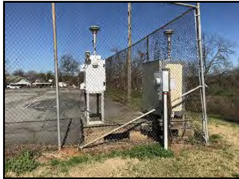
2 View of two sampling stations observed inside the tennis courts.
