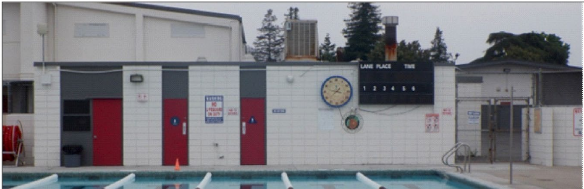
View of the southwest side of the existing pool house and restroom facilities.
