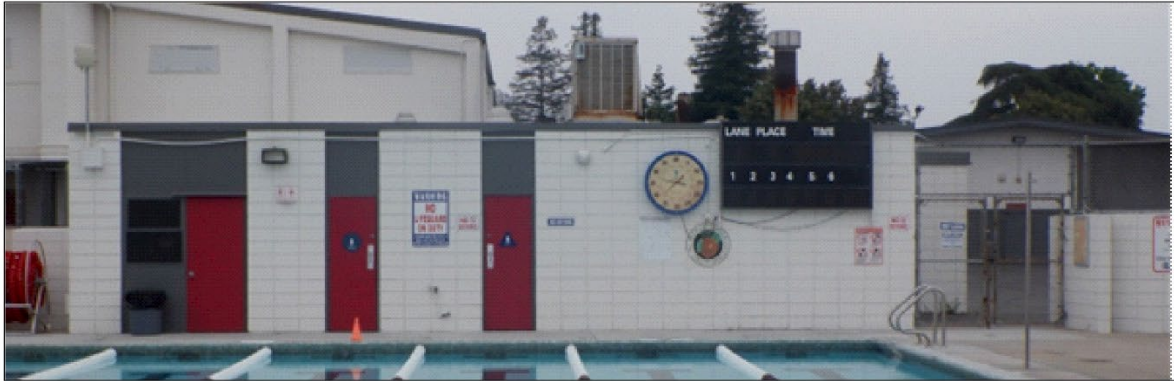
View of the southwest side of the existing pool house and restroom facilities.
