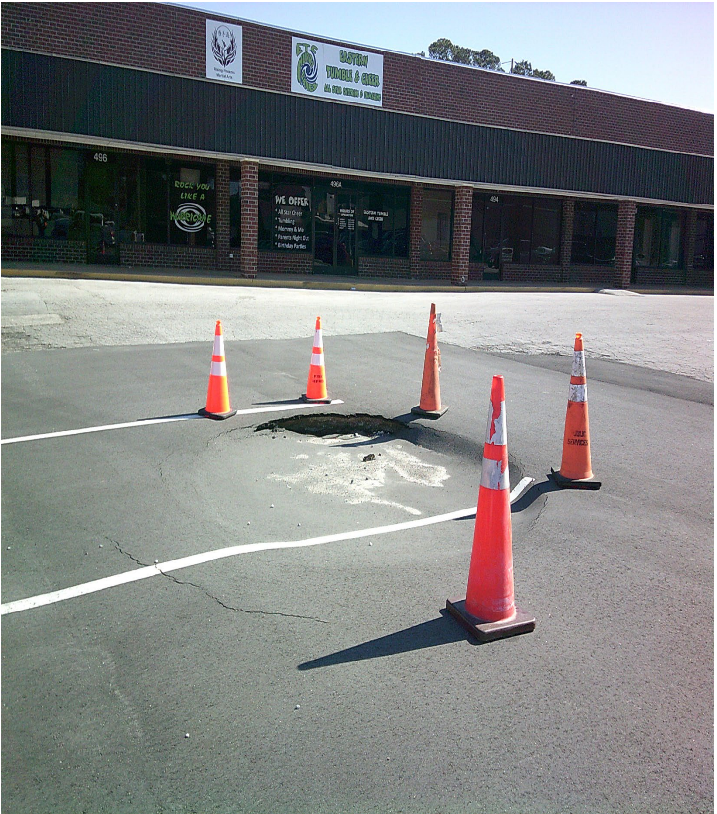
Figure 3: Pic of the work area
