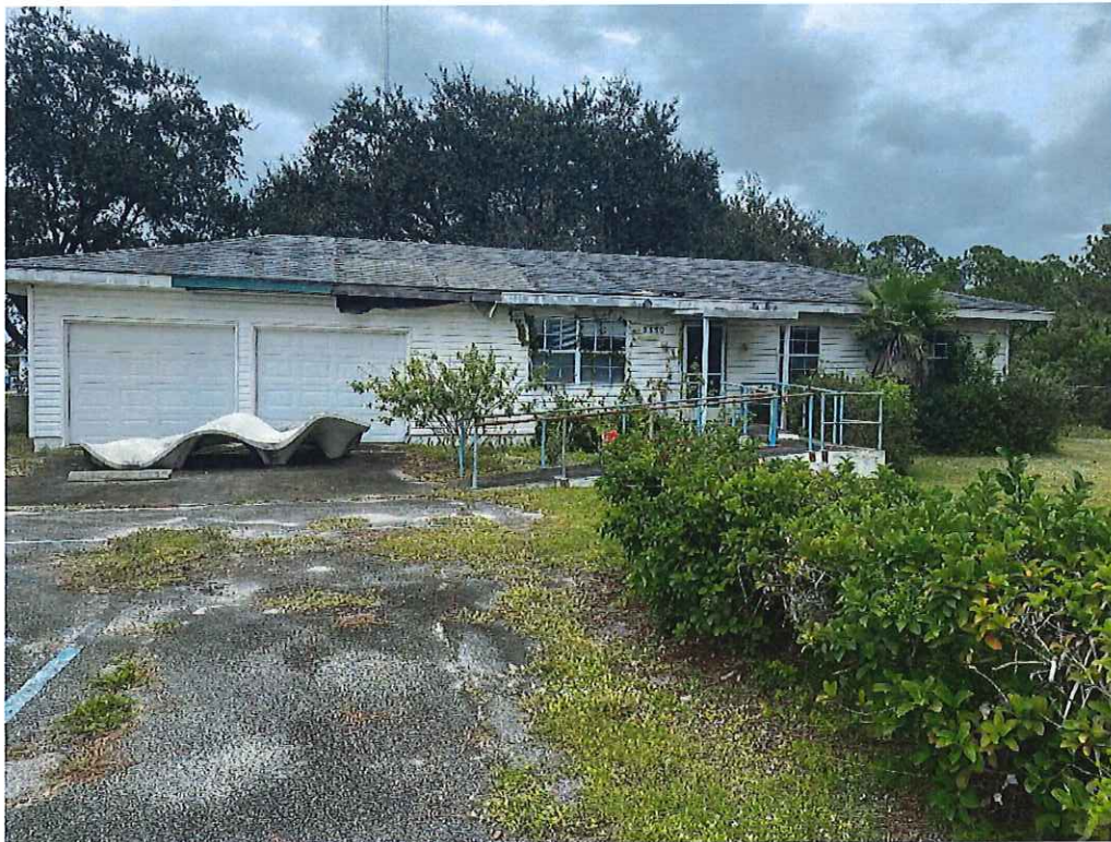
Looking North at Office Building
