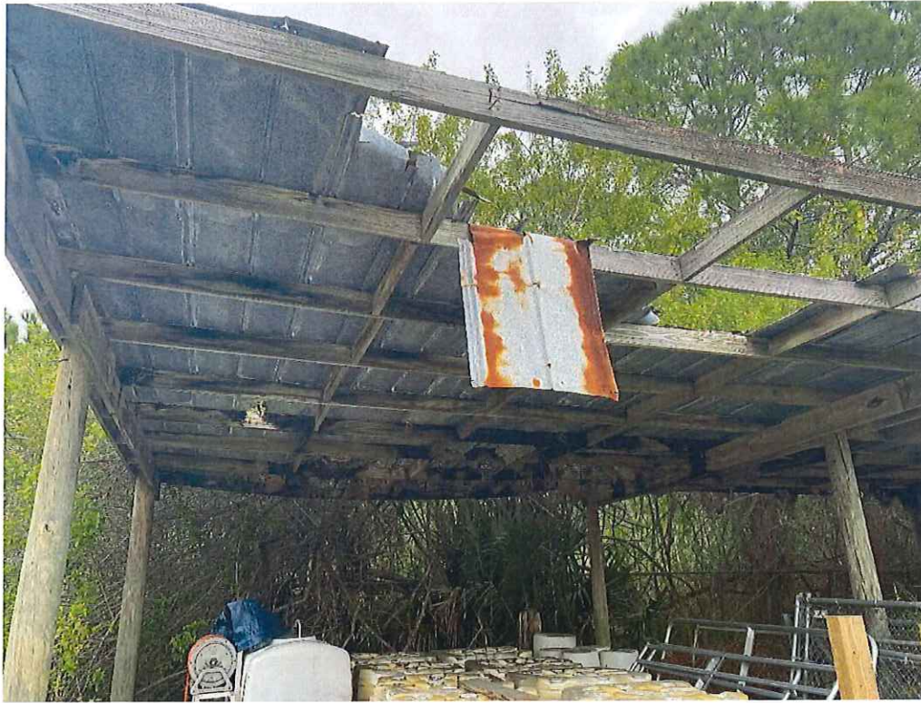
No Suspect Asbestos Containing Materials, Metal Roof/Wood Support, Pole Barn
