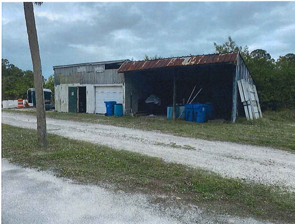
Looking Northeast at Old Shop Building
