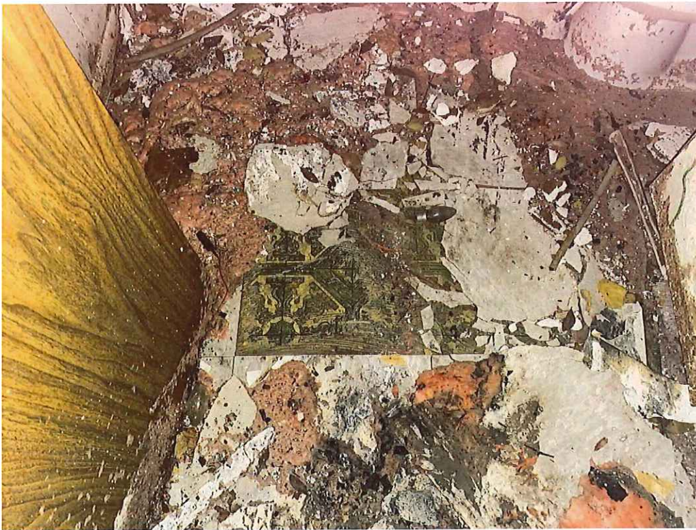
Sheet Flooring (Green), Bathroom, Closet at Kitchen, Office Building
