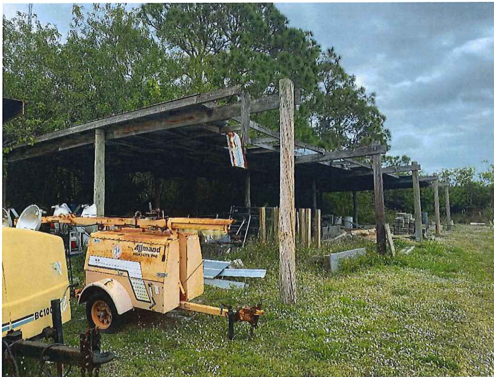
Looking Northeast at Pole Barn
