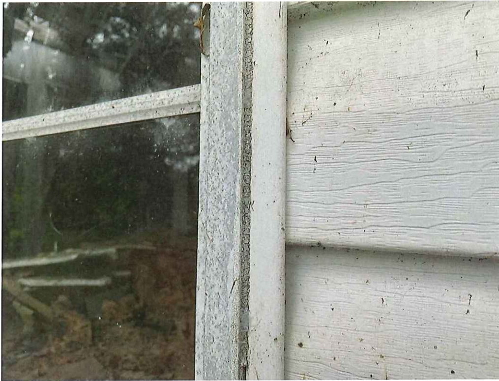
Window Caulking, Throughout Office Building
