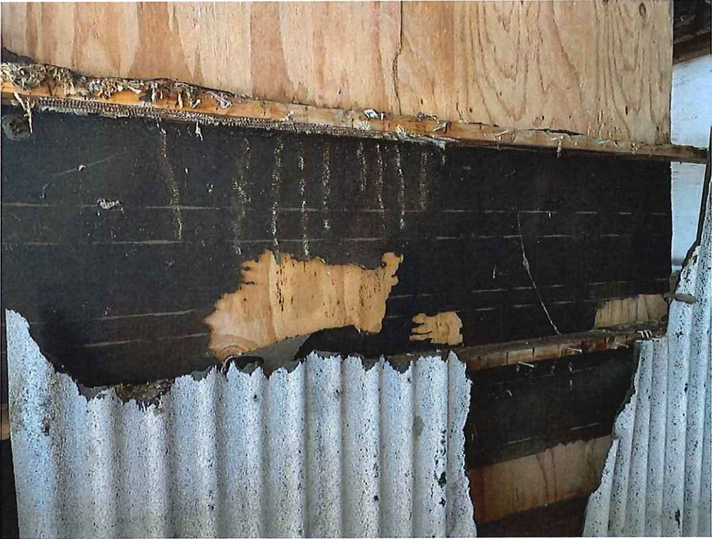
Feltpaper Behind Corrugated Siding, Old Shop Bulding
