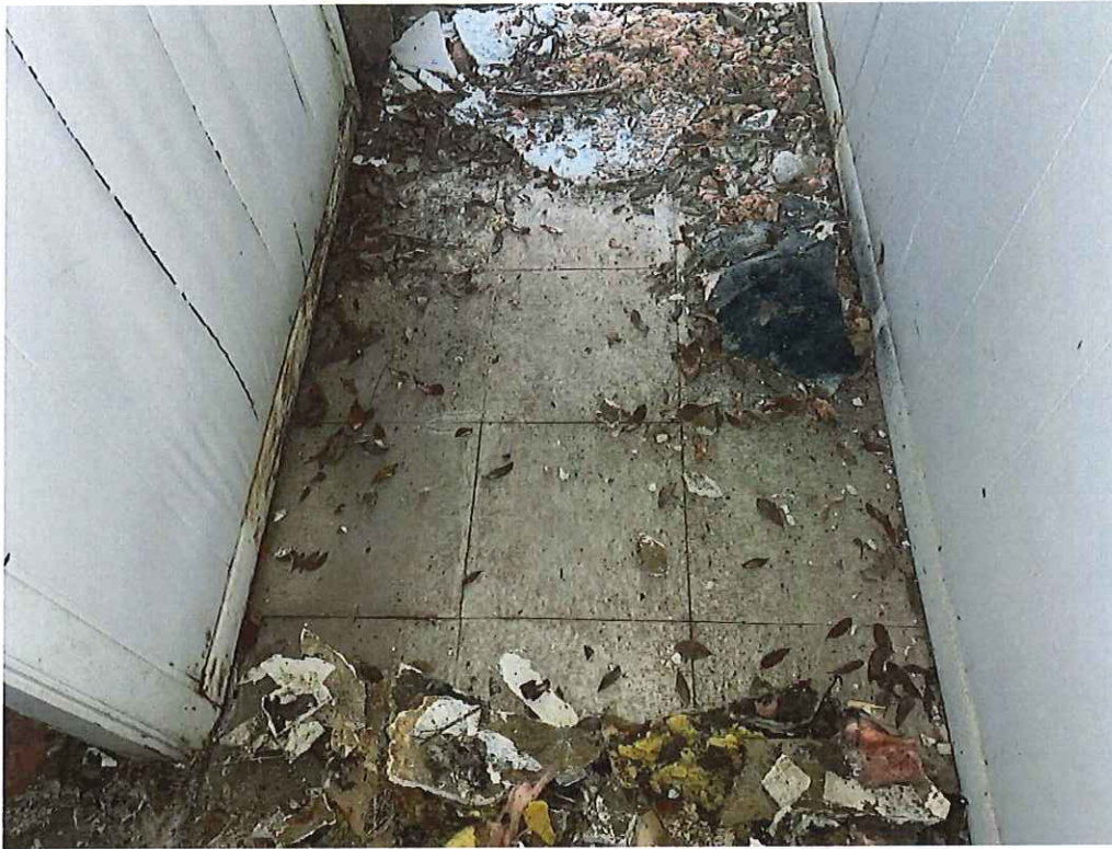
12" x 12" Floor Tile (Beige), Throughout Office Building
