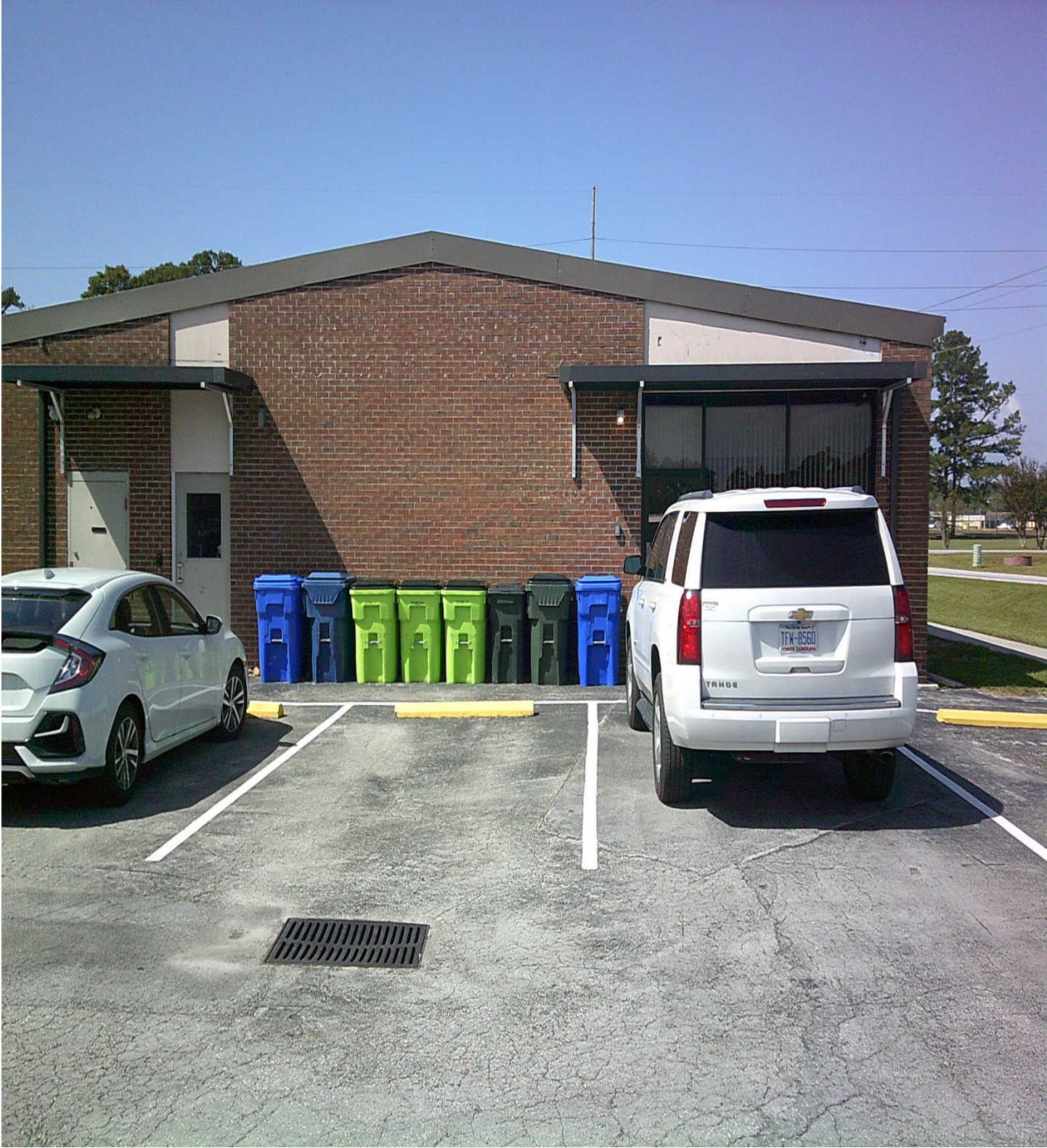
Figure 4: East Side of the Building
