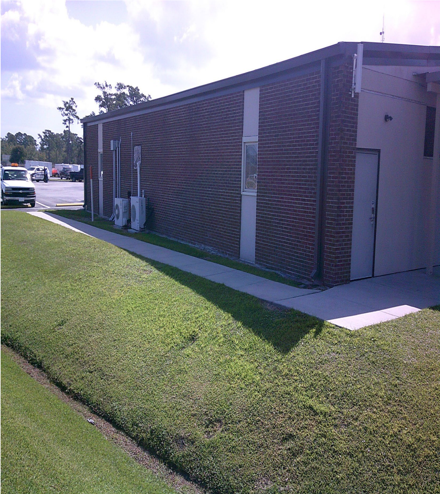
Figure 2: North Side of Building
