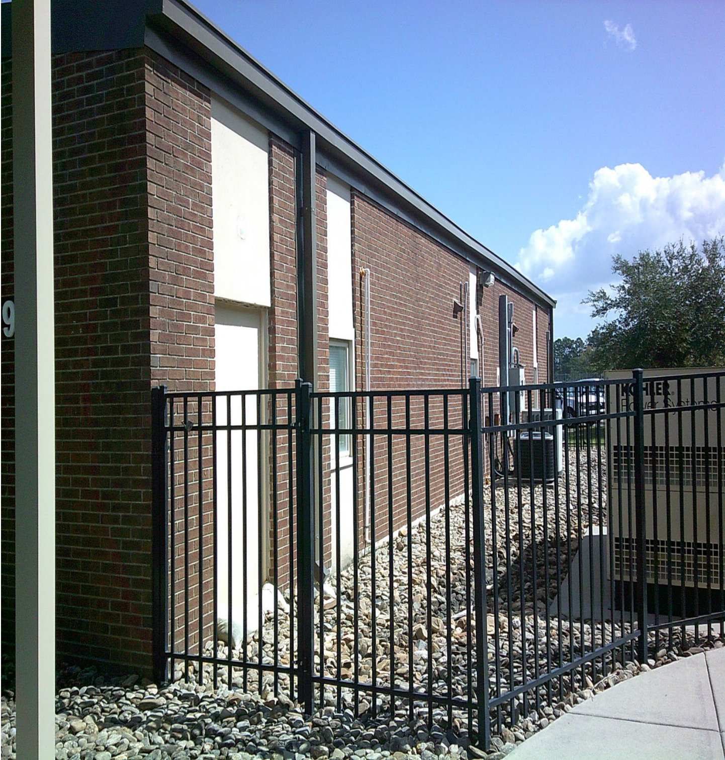
Figure 3 South Side of Building
