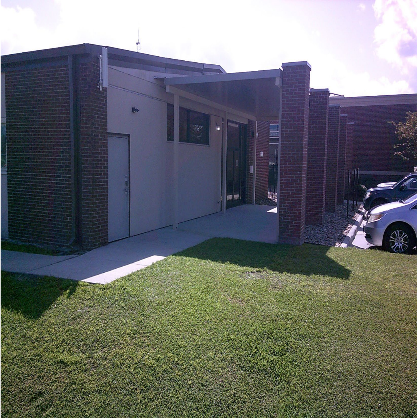
Figure 1: Front of Building / West Side
