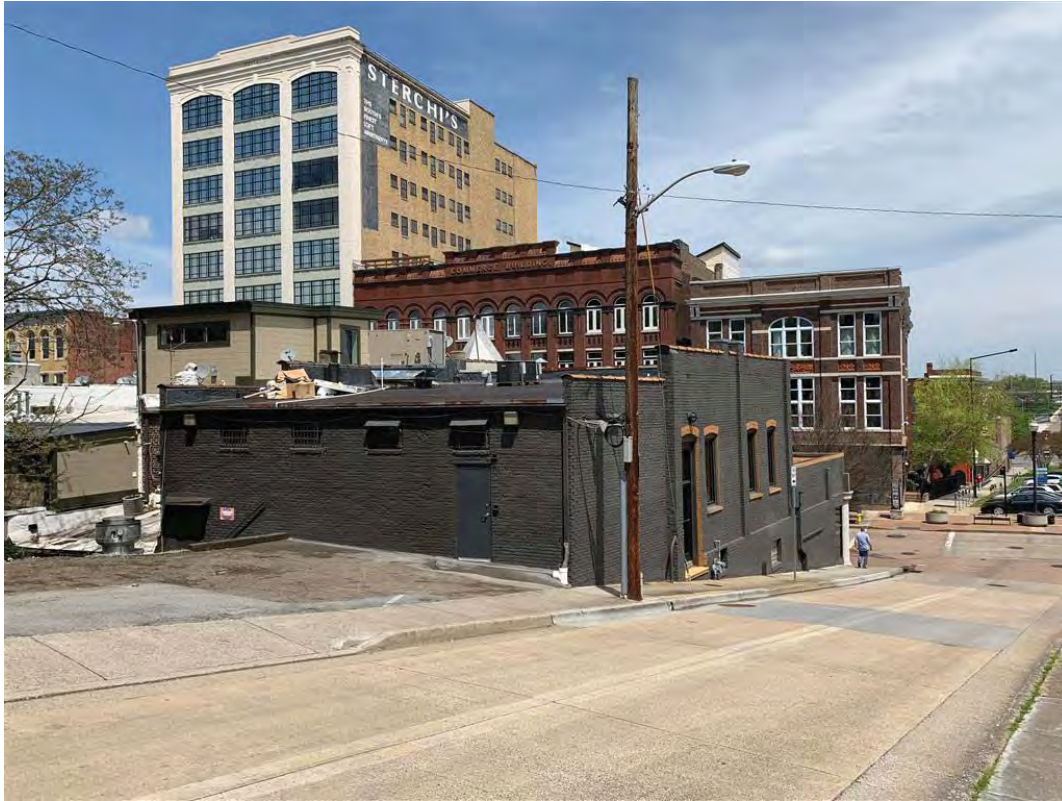
Photograph 5: Vacant commercial building across West Vine Avenue to the north of the Property
