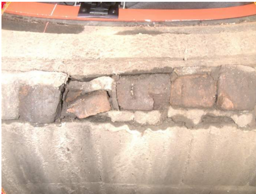
1837c_166883a2-6c9f-44dc-8d3b-993be20f6dc6_f4da2fc8-9b38-41b2-883b-1d13218a253a_P11.jpg, 00:00:00, 0.66 Displaced Brick from 6 o'clock to 8 o'clock
