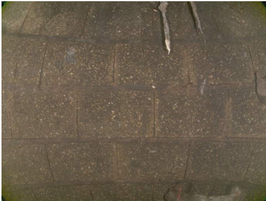
1838_4d464b94-a957-4557-a7ae-8bb14bf4d783_2af9f40c-8e6b-4a28-8936-9ca041e50edf_P11.jpg, 00:00:23, 4.86 Deposits Attached Ragging, 5% of cross sectional area from 6 o'clock to 8 o'clock, within 8 inch
