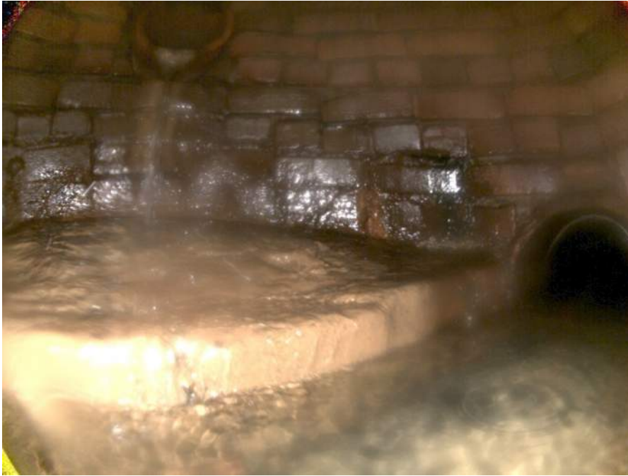
1830_f8e692ed-45a5-4111-be6d-dbb6437dd8b2_09a3541c-4a16-43e5-a383-d82113518f21_P11.jpg, 00:00:40, 8.82 Deposits Settled Fine, 15% of cross sectional area from 12 o'clock to 12 o'clock, within 8 inch
