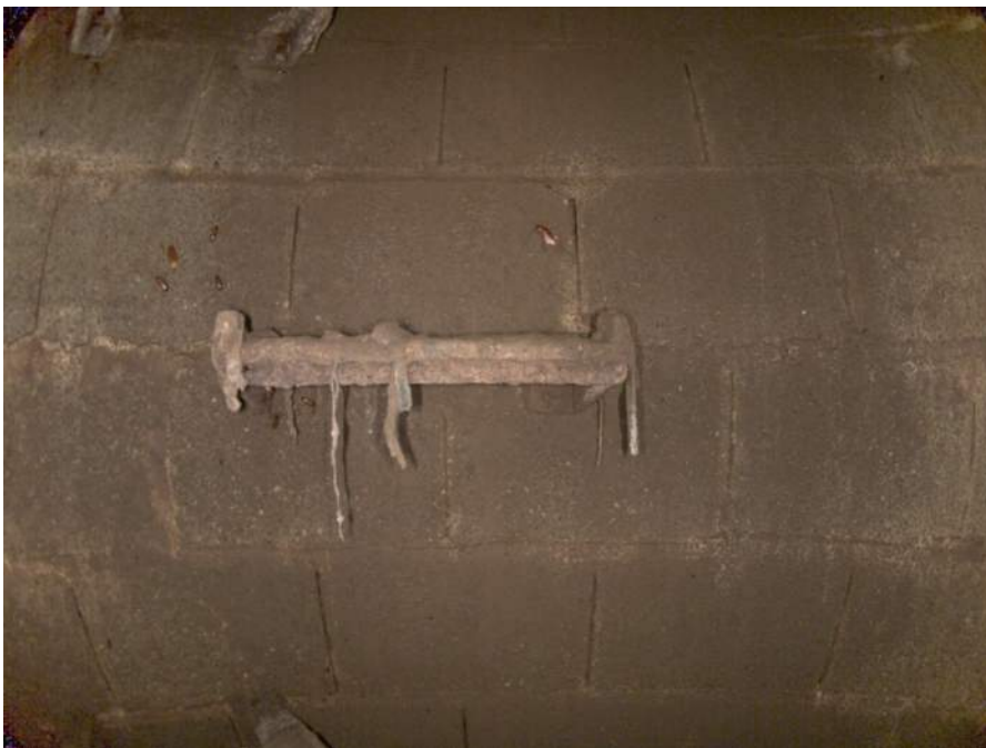
1841a_7e3e94ed-5602-4c81-88a8-bfb0bb428782_daacd105-63d3-4004-8c79-a586eef84f9f_P11.jpg, 00:00:30, 7.10 Deposits Attached Ragging, 5% of cross sectional area from 8 o'clock to 12 o'clock, within 8 inch
