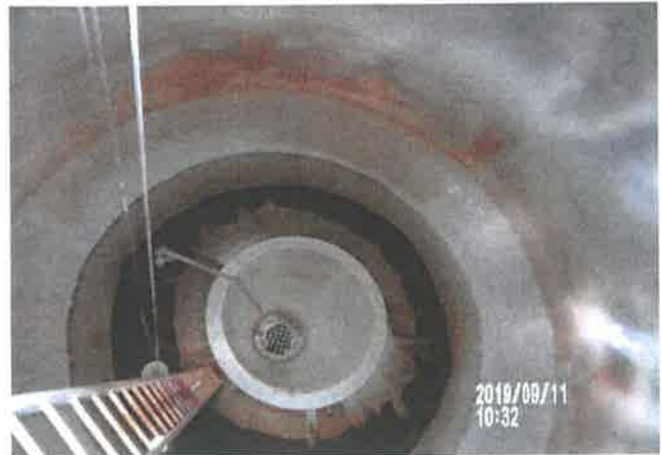
Interior During Washout
