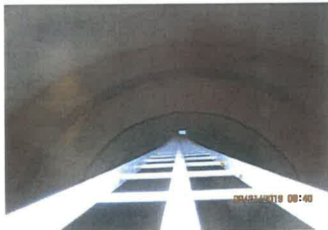
Interior Access Ladder
