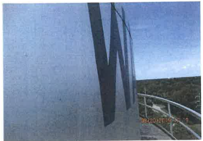
Exterior Sidewall Coating
