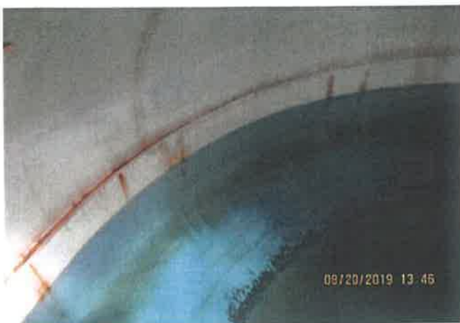
Interior Sidewall/Roof Coating
