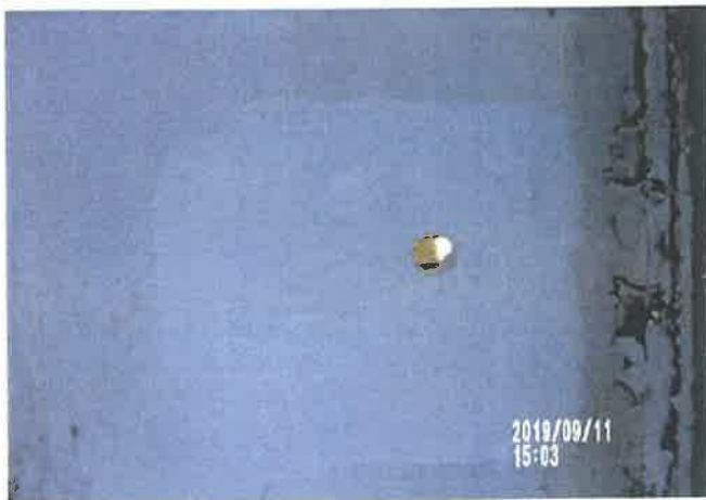
Balcony Weep Holes Drilled and Coated
