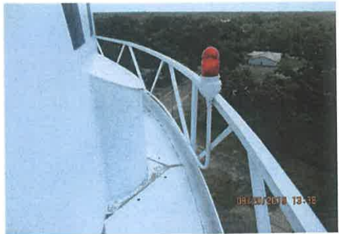
Balcony and Handrail
