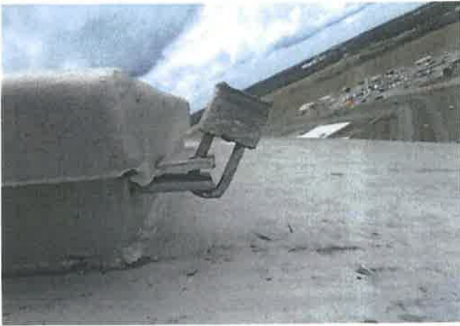
Locked Access Hatch
