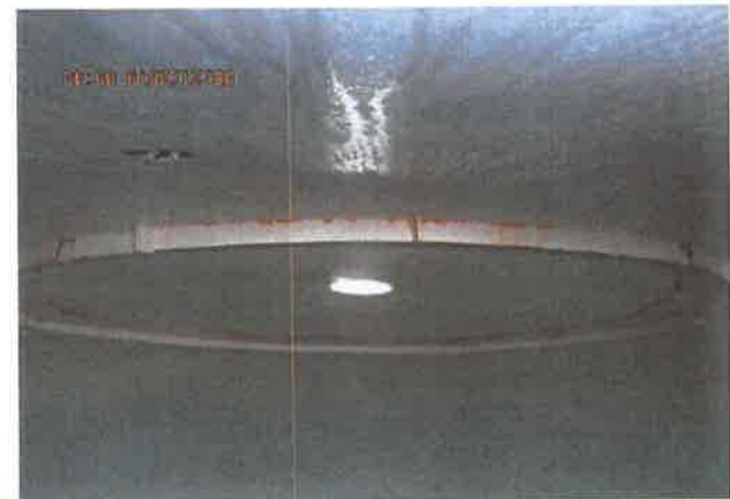
Interior Roof Structure
