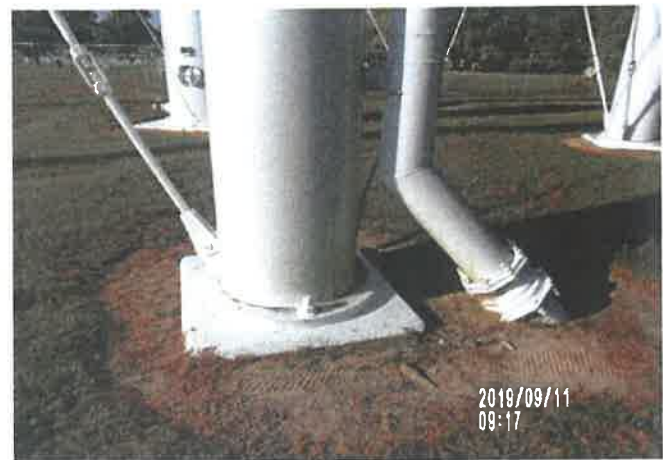
Exterior Leg Base and Overflow Coating
