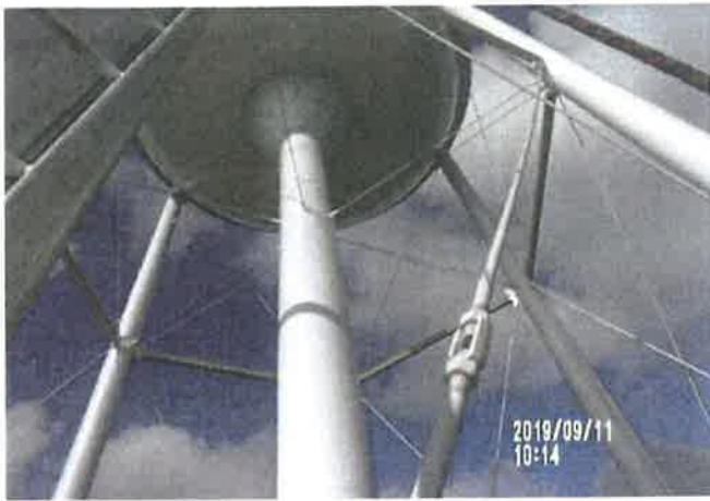
Exterior Riser Coating
