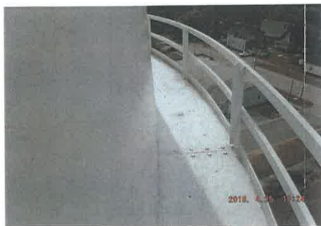
Balcony and handrail
