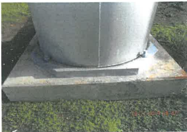
Exterior Riser Base Coating
