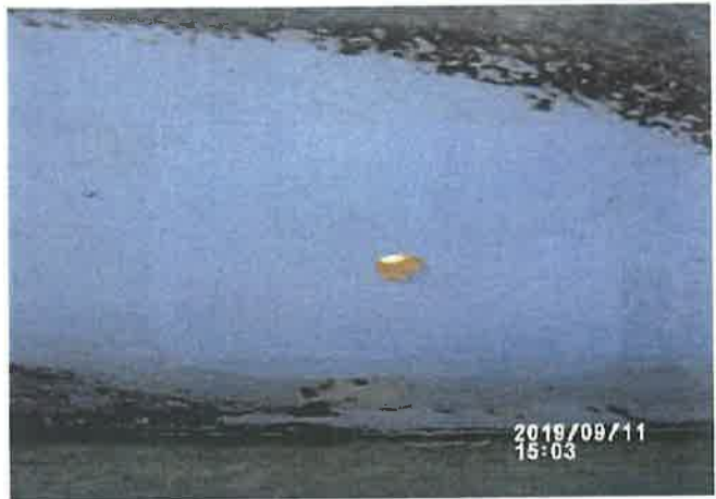
Balcony Weep Holes Drilled and Coated
