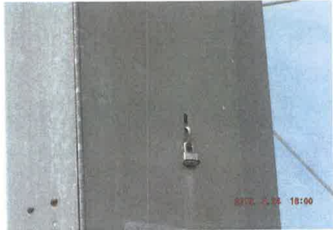
Ladder gate locked
