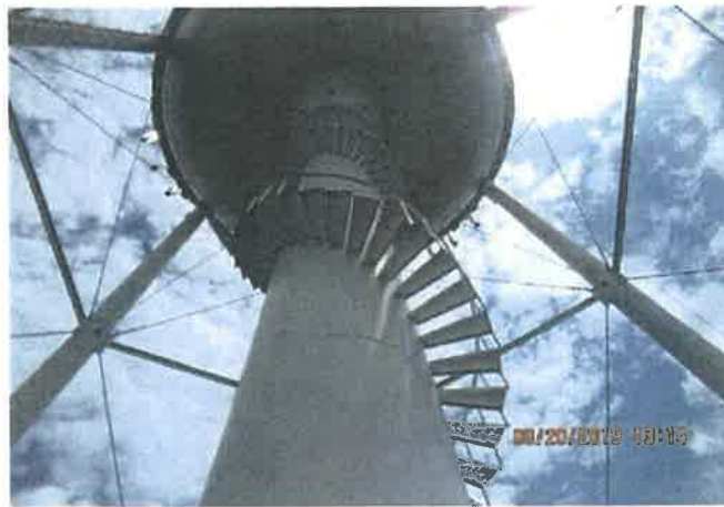
Exterior Under Belly Coating
