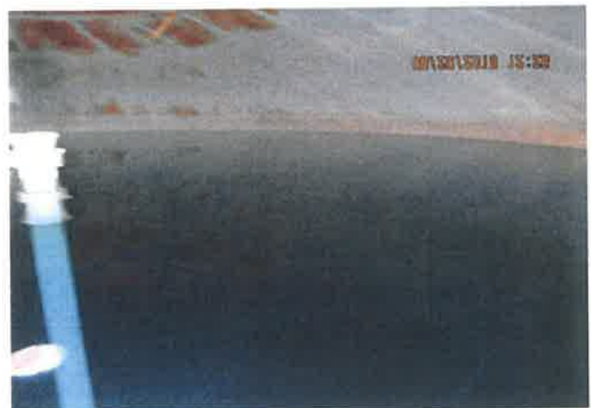
Interior Sidewall/Roof Coating
