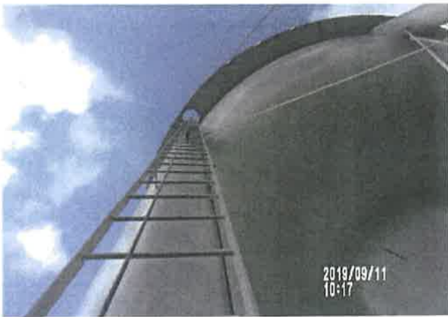
Cable Safety Climb on Access Ladder
