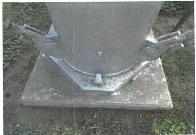
Exterior Leg Base Coating
