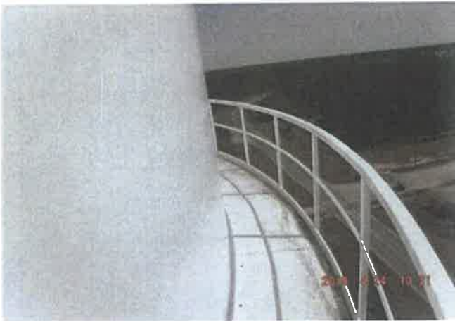
Balcony and handrail
