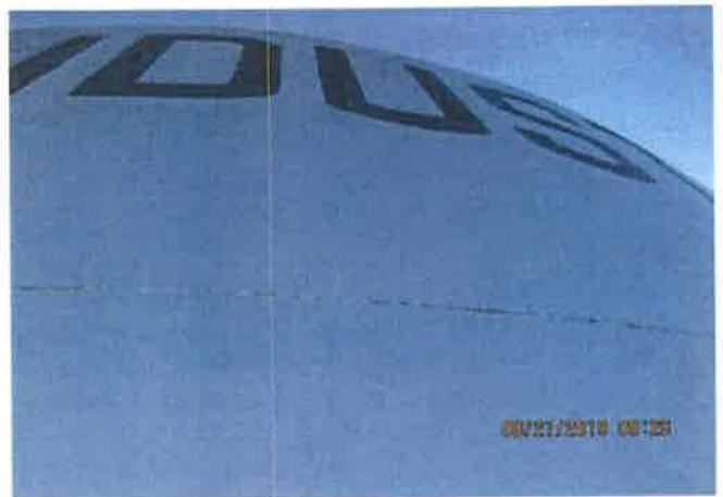
Exterior Logo and Sidewall Coating
