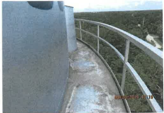
Balcony and Handrail
