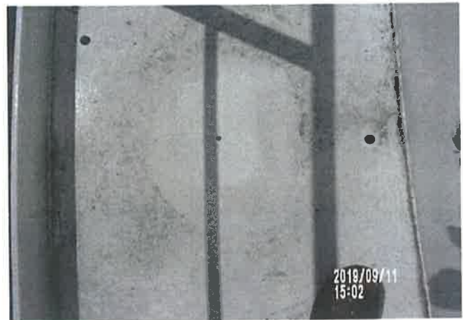
Balcony Weep Holes Drilled and Coated
