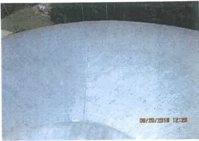
Exterior Roof Coating
