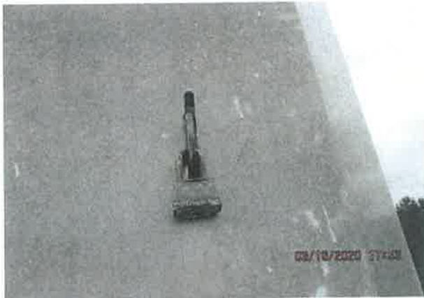
Ladder gate locked
