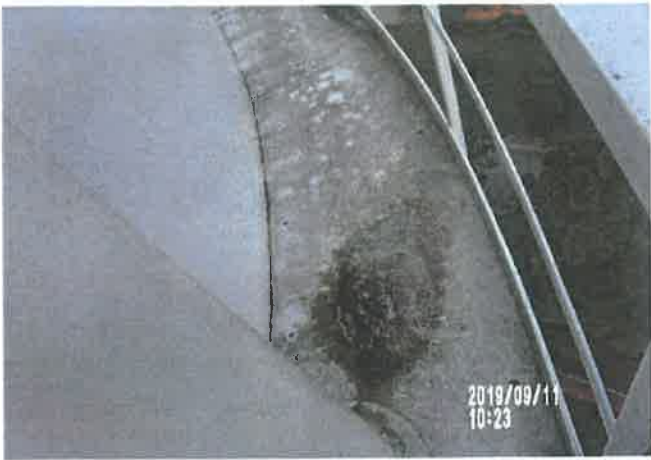
Balcony Before Repairs
