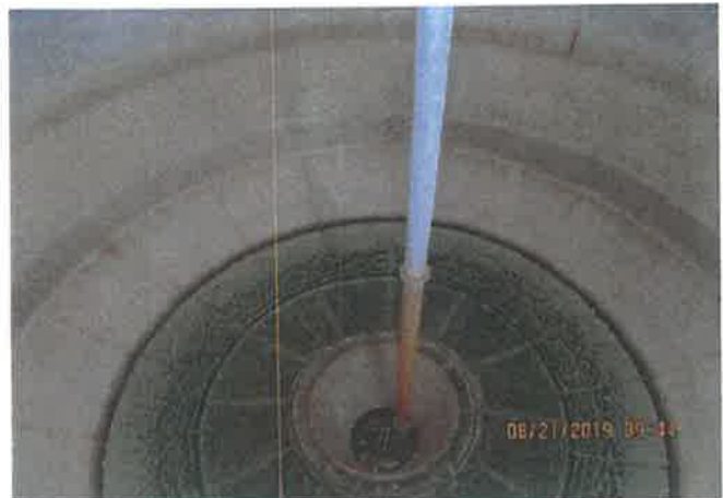
Interior During Washout
