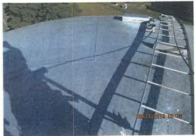
Exterior Roof Coating
