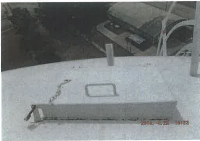
Roof access hatch
