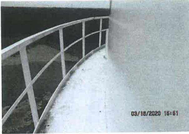
Balcony and handrail
