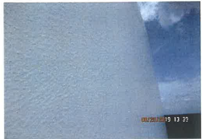
Exterior Sidewall Coating
