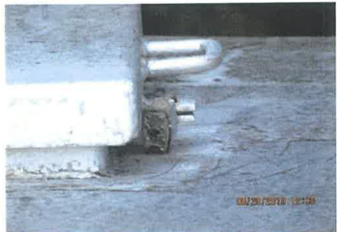
Wet Interior Access Hatch Locked
