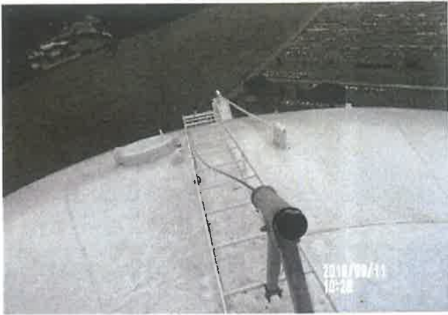
Exterior Roof Coating
