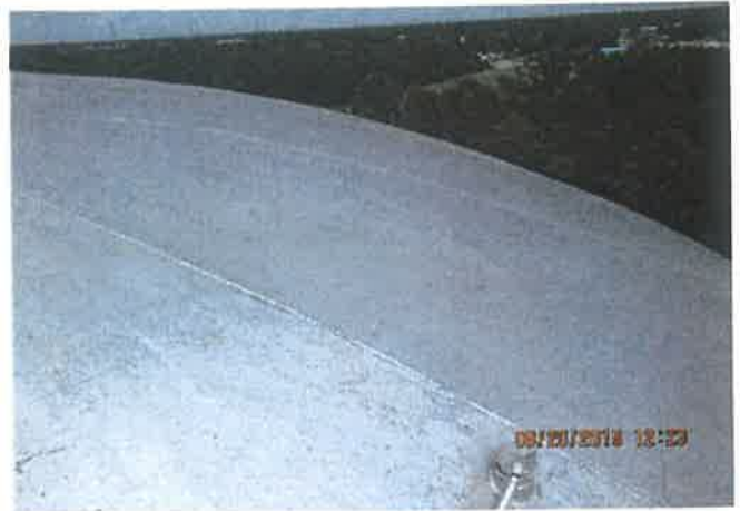
Exterior Roof Coating
