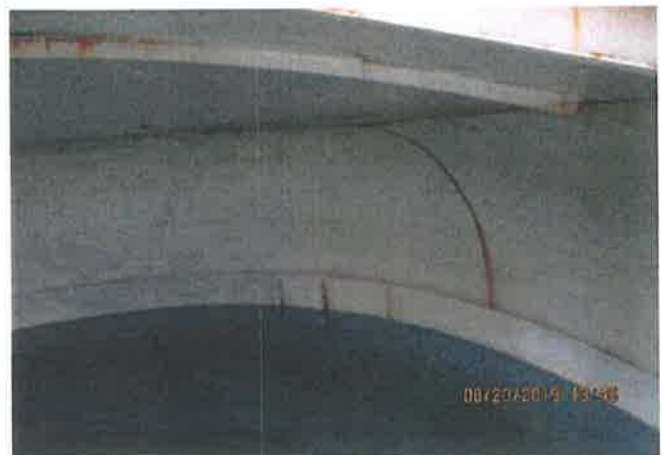
Interior Sidewall/Roof Coating
