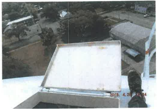
Roof access hatch
