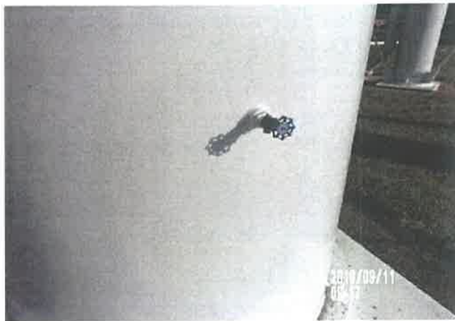
Exterior Riser Base Coating
