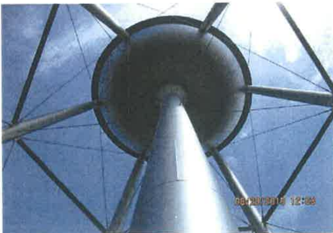
Exterior Under Belly Coating
