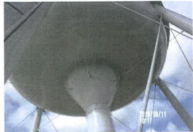
Exterior Under Belly Coating
