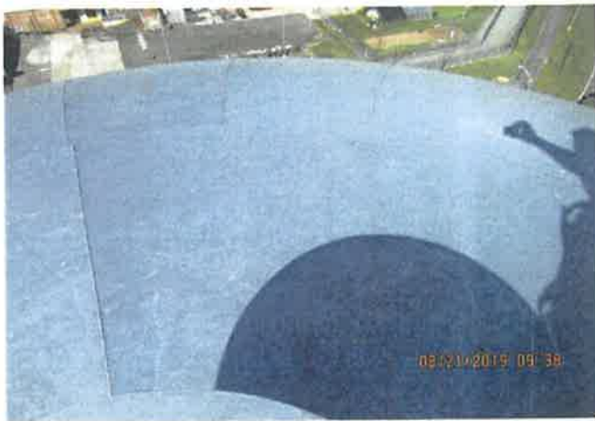
Exterior Roof Coating
