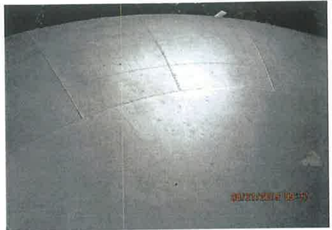
Exterior Roof Coating
