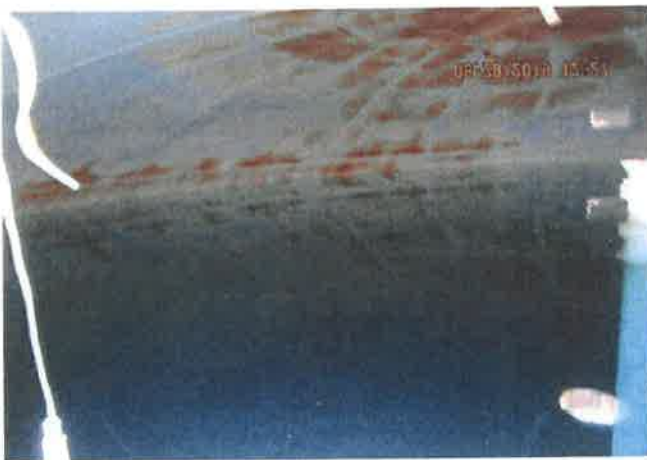
Interior Sidewall/Roof Coating
