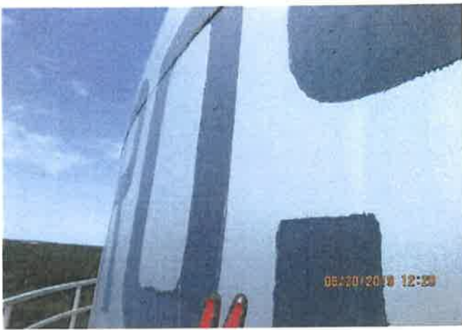
Exterior Sidewall Coating
