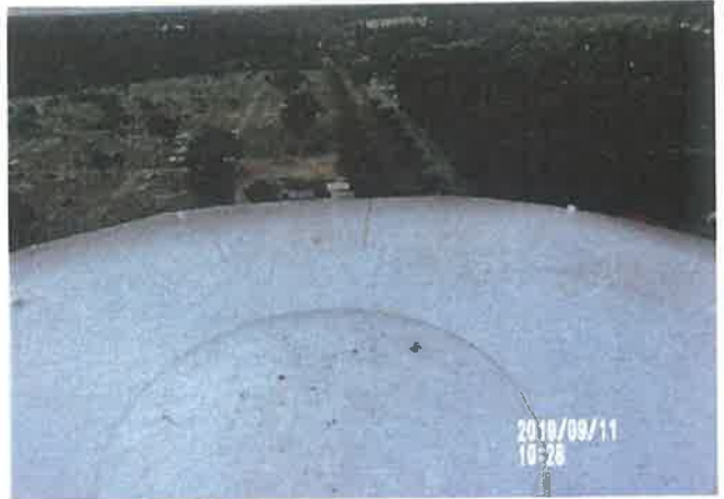
Exterior Roof Coating
