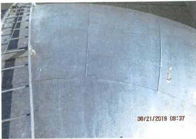
Exterior Roof Coating
