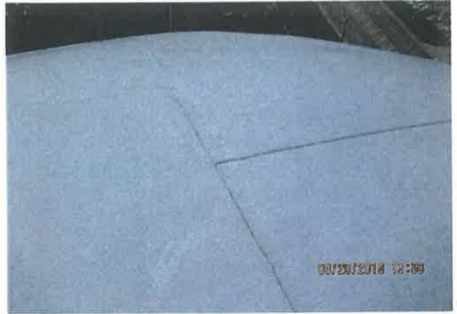
Exterior Roof Coating
