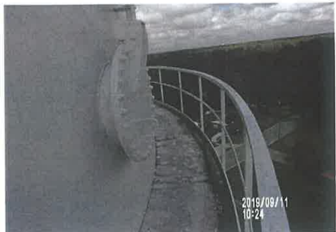
Davit Arm Sidewall Manway
