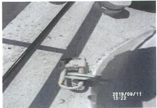
Locked Access Hatch
