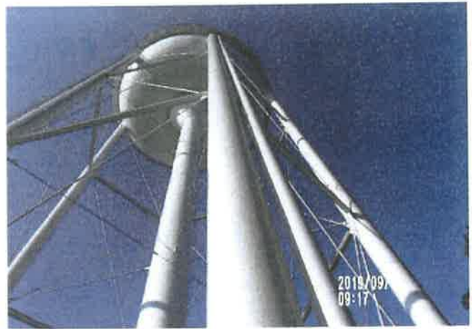
Exterior Leg and Overflow Pipe Coating
