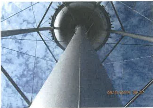
Exterior Under Belly and Riser Coating
