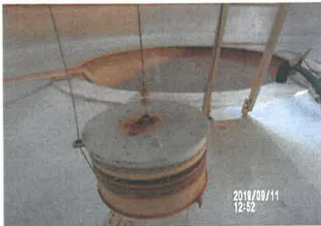
Float Repaired During Washout
