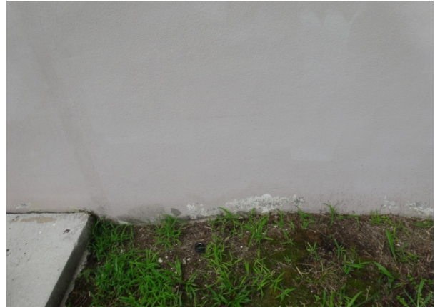
Photo 8 Paint degradation
