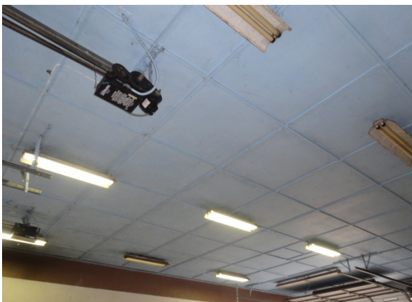
Photo 11 Plywood ceiling in apparatus bay – no evidence of moisture intrusion
