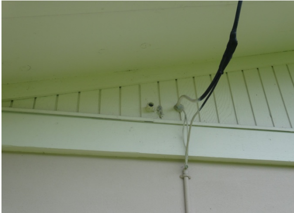
Photo 7 Open conduit into attic
