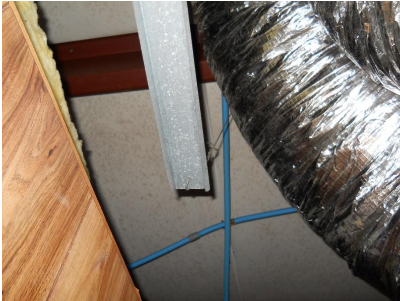
Photo 1: Microbial growth on vinyl-faced insulation within Office 207.
