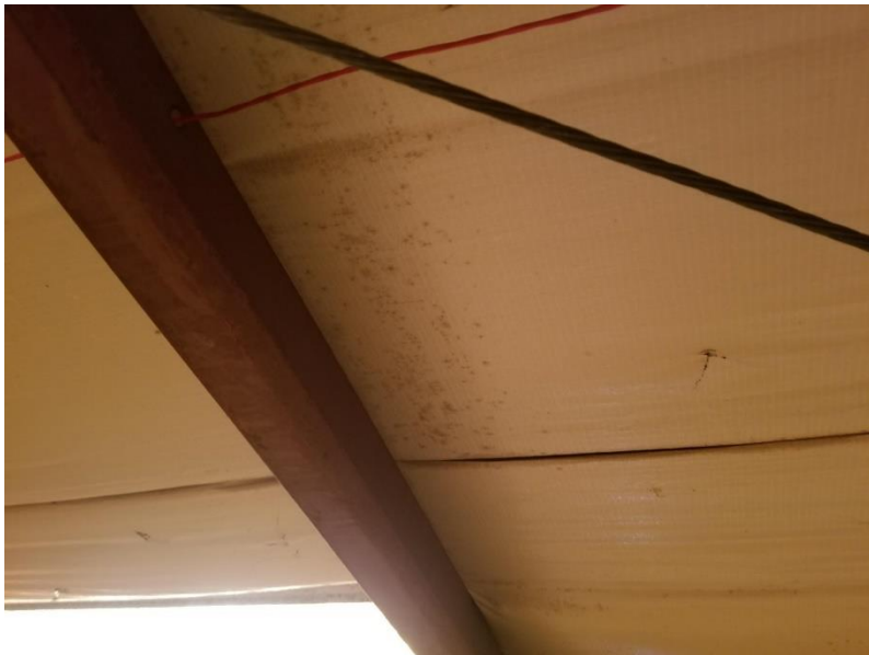
Photo 3: Microbial growth on vinyl-faced insulation within the rear mezzanine.
