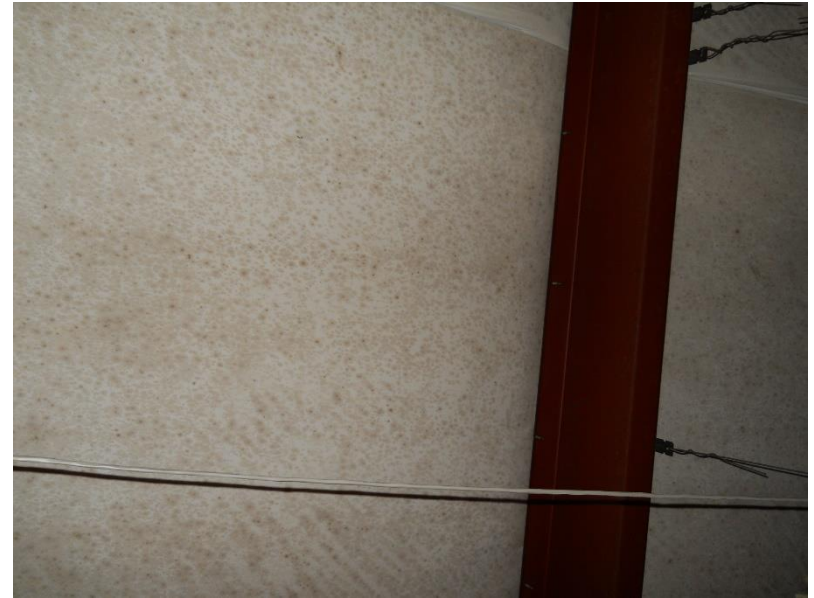
Photo 2: Microbial growth on vinyl-faced insulation within Office 201.
