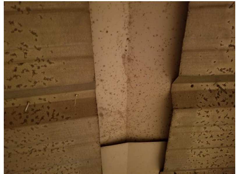
Photo 4: Microbial growth on metal crown flashing within the rear mezzanine.
