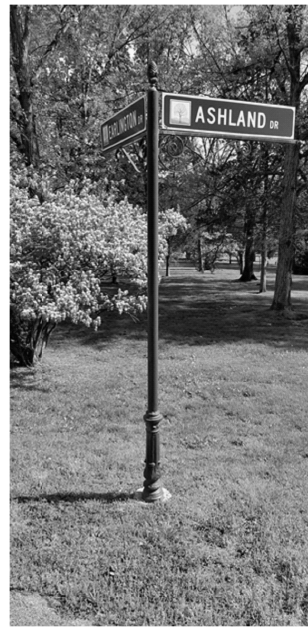
SP-2: DECORATIVE STEEL SIGN POLE WITH BASE (STREET NAME SIGN) NOT TO SCALE
