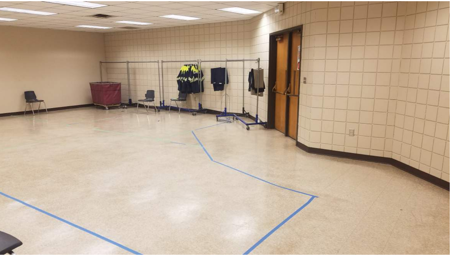
5 PHOTO NOT TO SCALE B-1 EXISTING CONDITIONS
