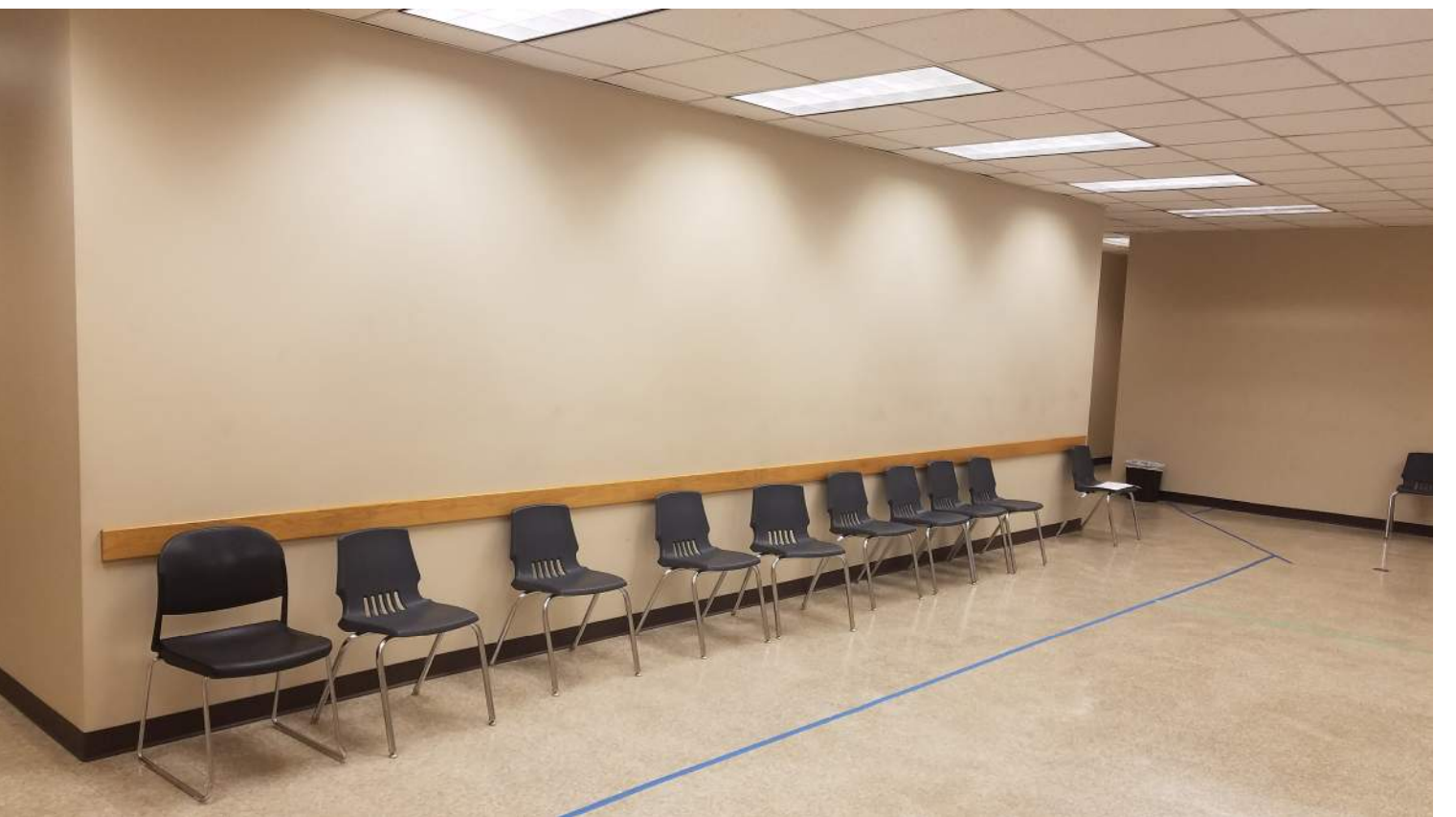
3 PHOTO NOT TO SCALE B-1 EXISTING CONDITIONS
