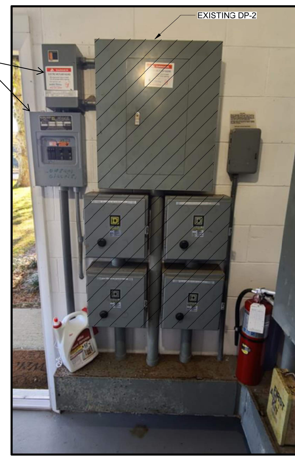
EXISTING ELECTRICAL ROOM - EAST WALL ELEVATION - DEMO
