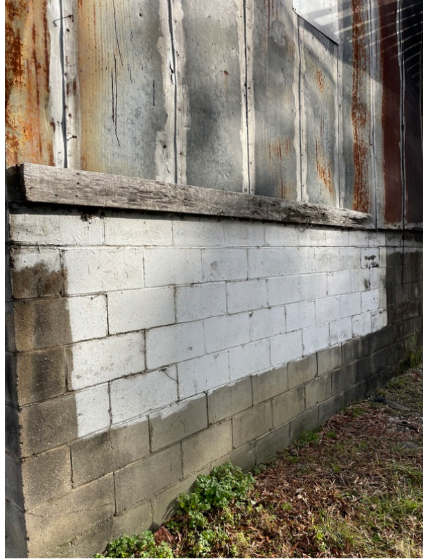
View of the asbestos-containing White/ Silver Exterior CMU Surfacing (HA 3-7)
