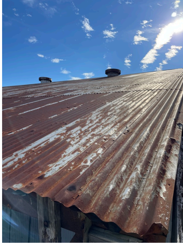
View of the asbestos-containing Silver Roof Paint (HA 4-2)
