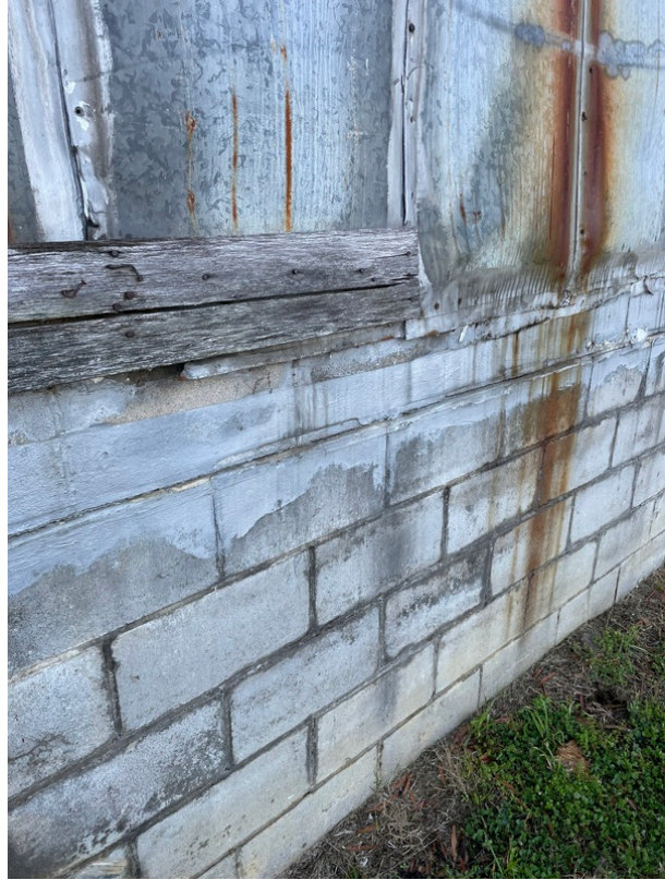
View of the asbestos-containing Silver Exterior CMU Surfacing (HA 3-5)
