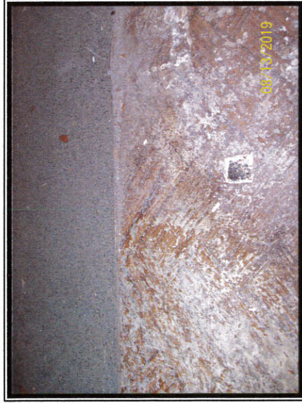
Photo #3 Asbestos Detected at >1% in Tan Floor Tiles under Parquet Sheet Flooring at Counter Area
