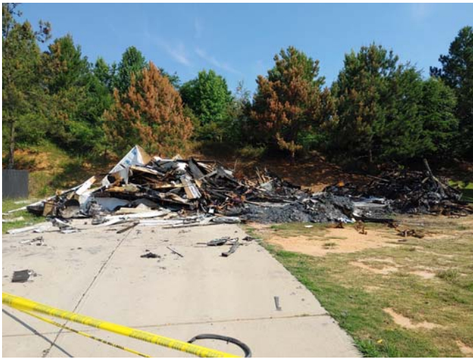
Photo 1 – Typical view of 213 Windigo Road in Spartanburg, South Carolina 29306
