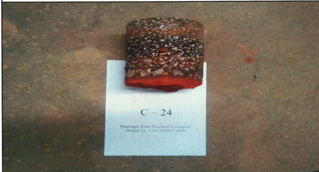
Photo 48: Pavement core C-24.
