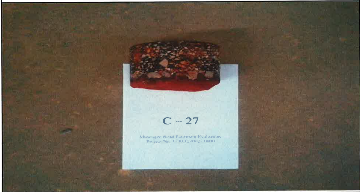
Photo 54: Pavement core C-27.
