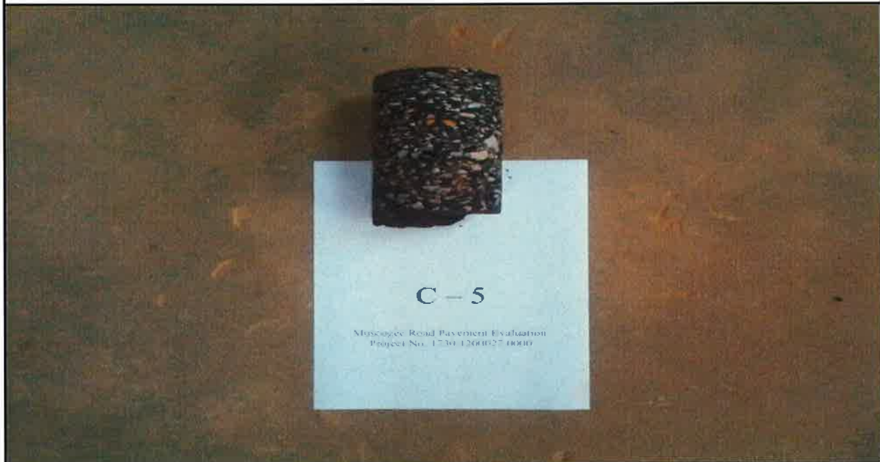
Photo 10: Pavement core C - 5.
