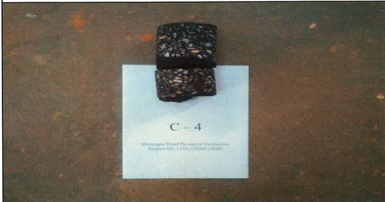
Photo 8: Pavement core C-4.
