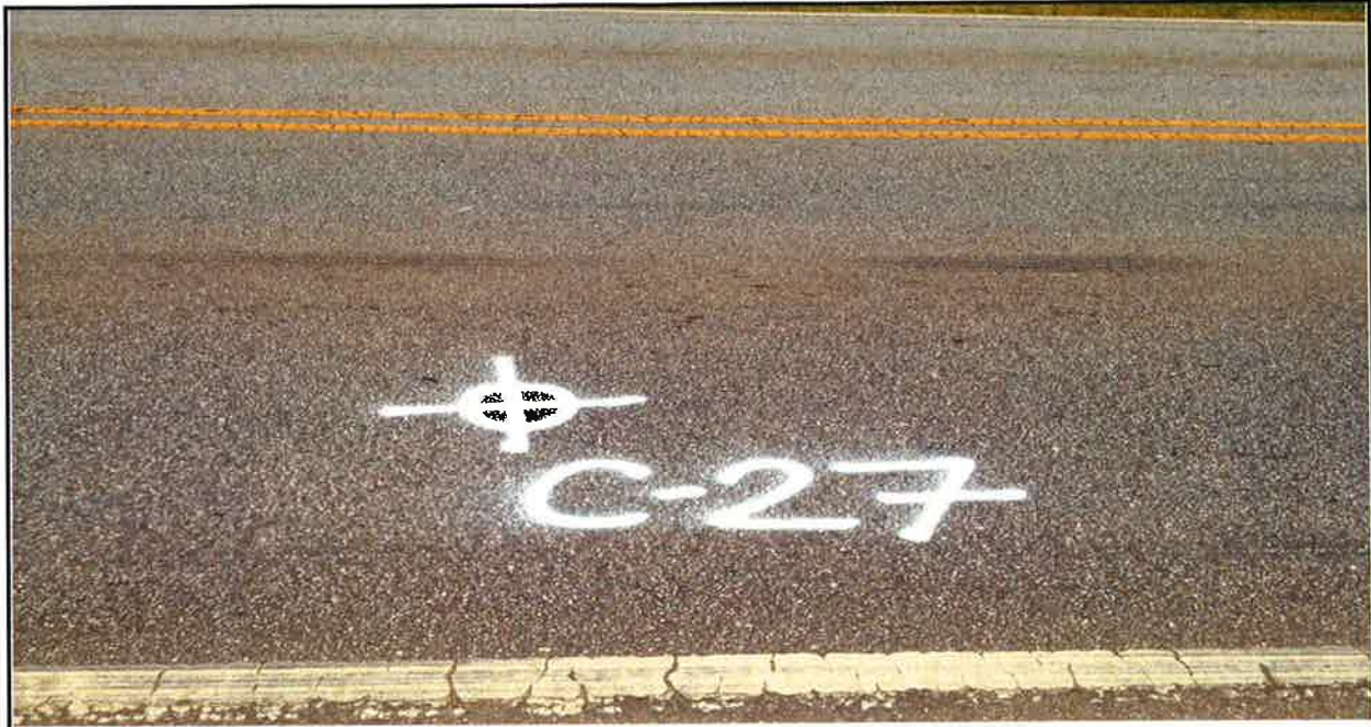
Photo 53: Minor rutting and weathering.
