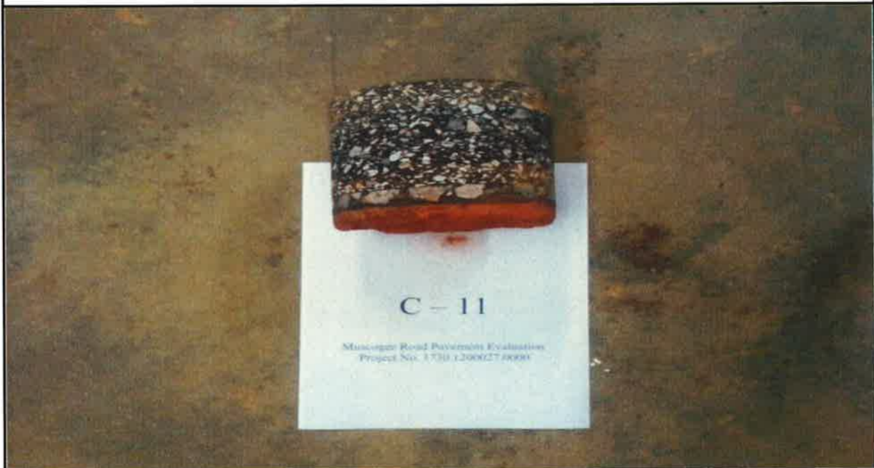
Photo 22: Pavement core C-11.
