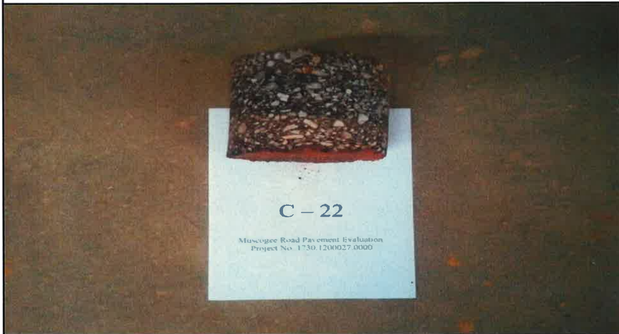
Photo 44: Pavement core C-22.
