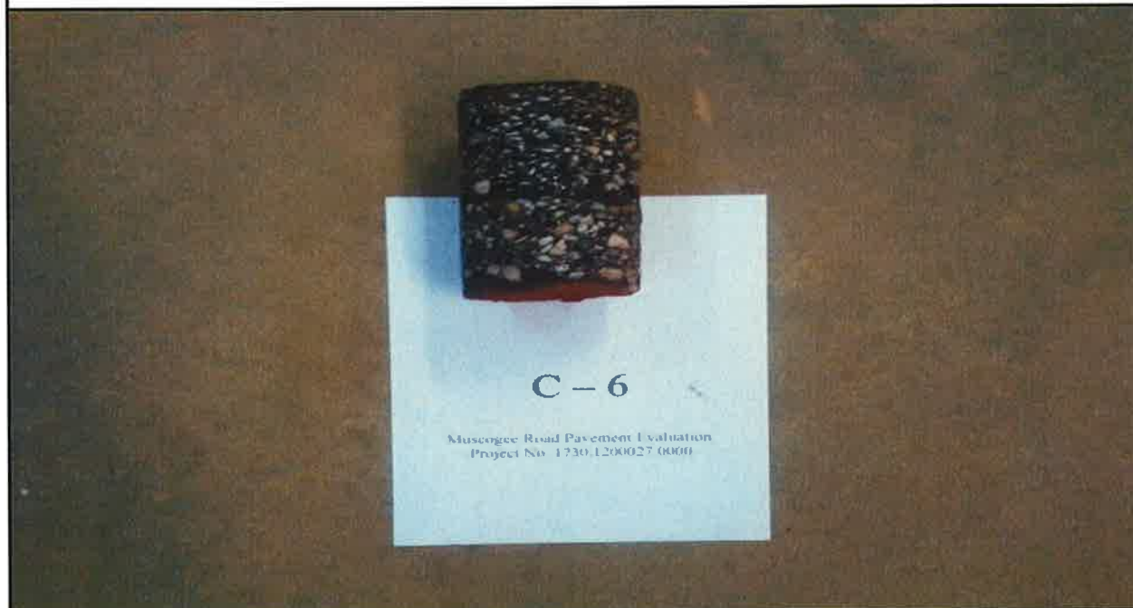
Photo 12: Pavement core C - 6.
