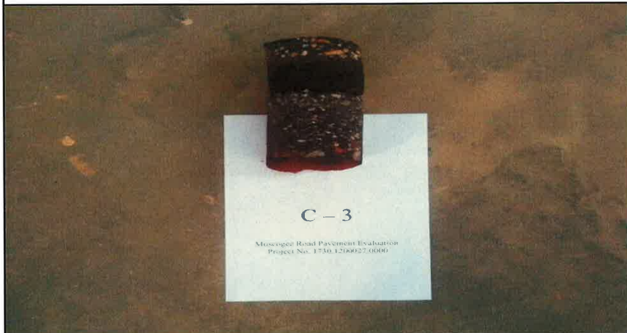
Photo 6: Pavement Core C-3.
