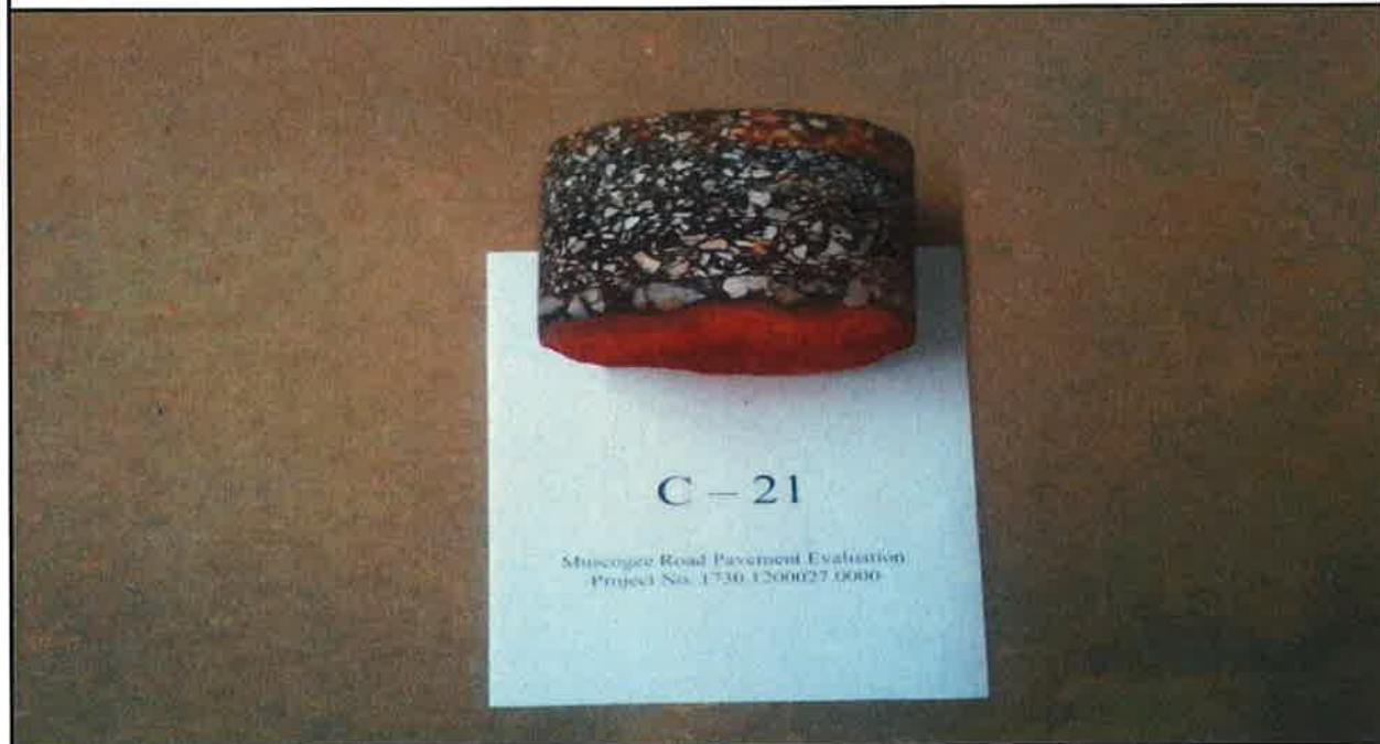
Photo 42: Pavement core C-21.
