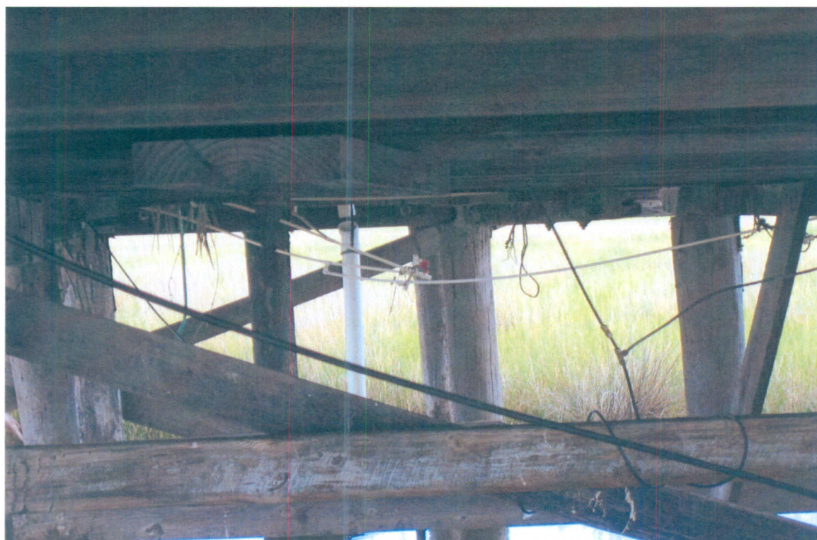
Pipe protruding from camp floor believed to be former sewer drop
