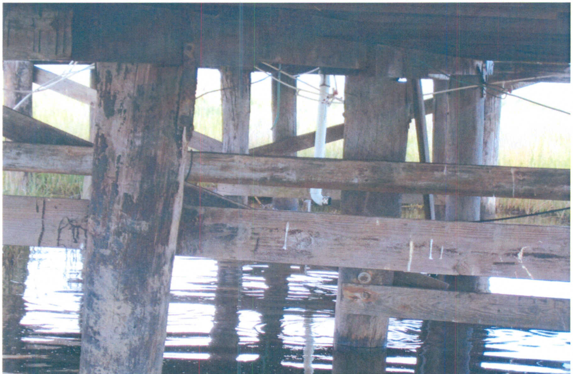
4 Pipe protruding from camp floor believed to be former sewer drop
