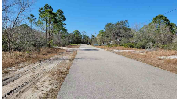
ADAM RD NW FACING NORTHWEST
