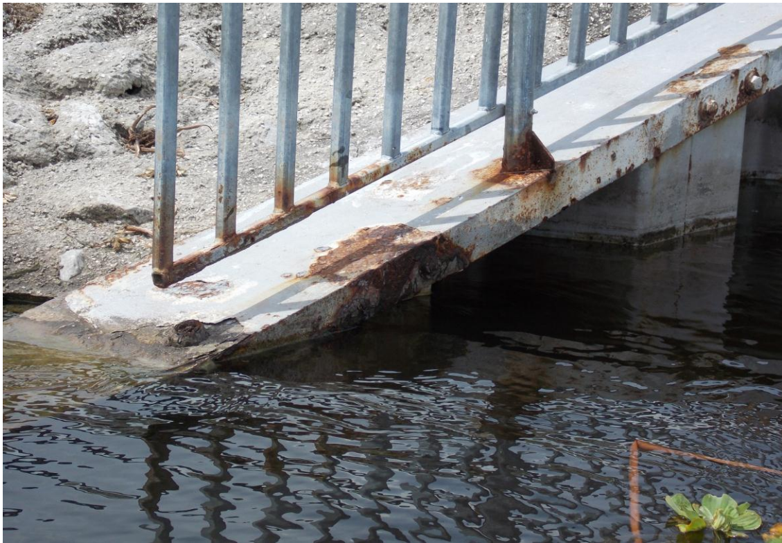
Upstream - South Wing Wall.
