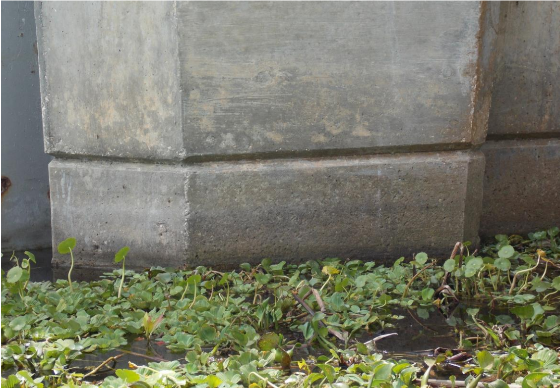
Upstream - South Structure Wall.
