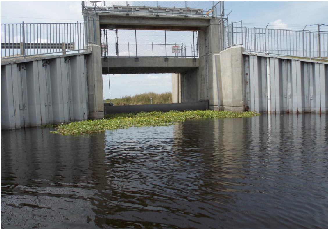
Upstream - Structure and Wing Walls.
