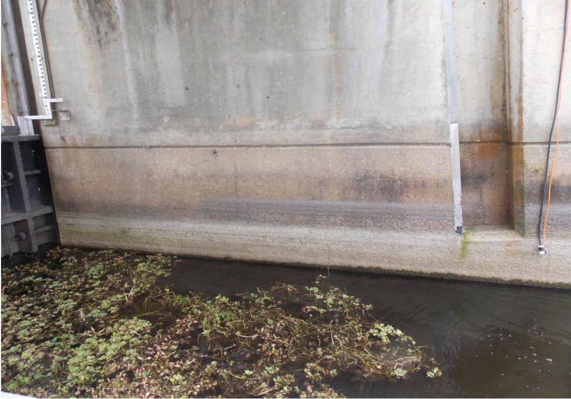
Downstream - South Structure Wall.
