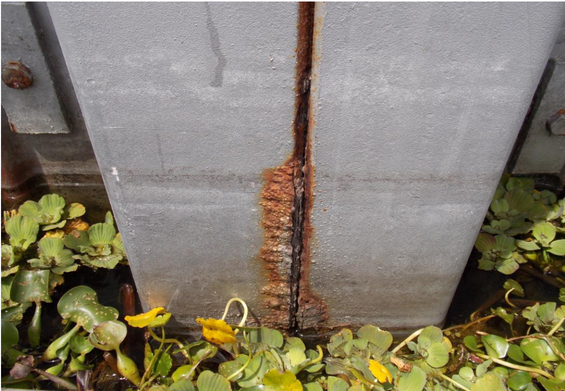
Upstream - North Wing Wall Corrosion at Joint.
