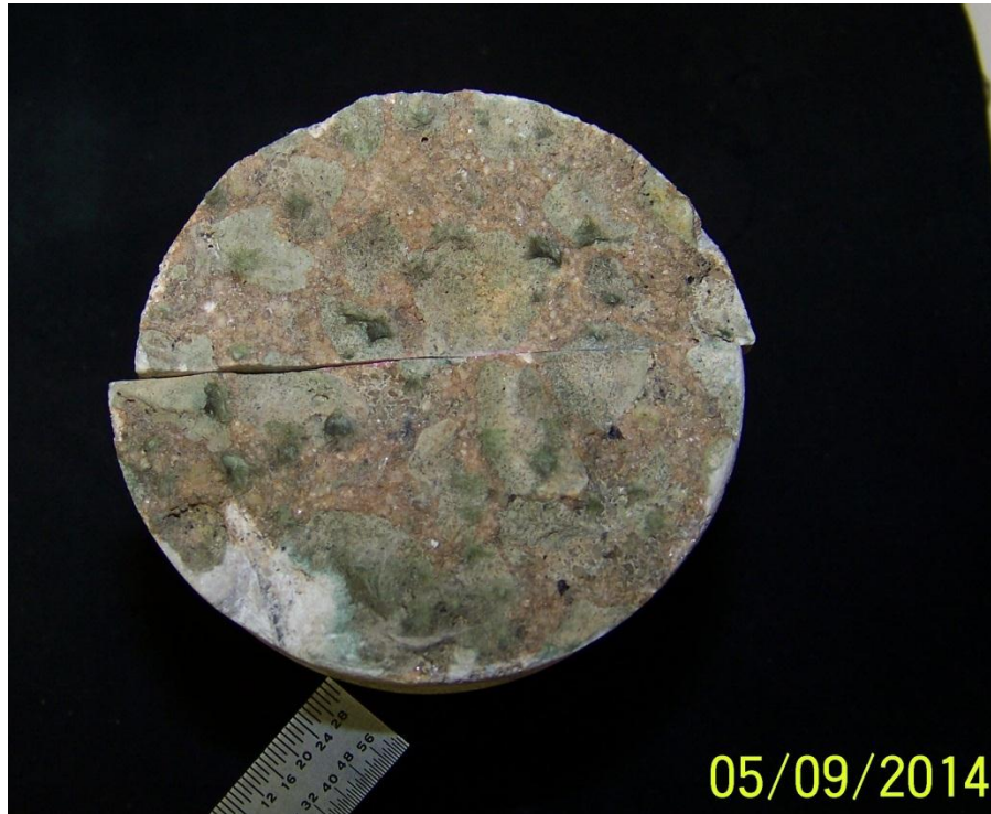
Photo 2 – Sample 1A – end view, note surface erosion.
