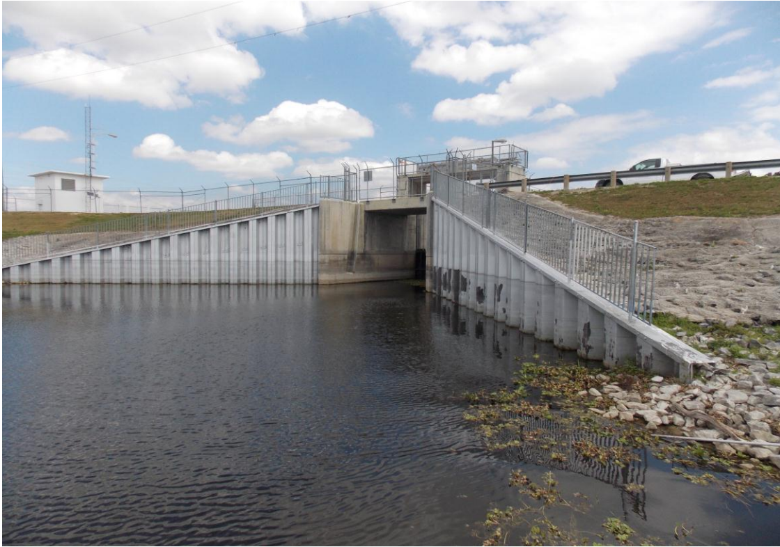
Downstream - View of Structure and Wing Walls.
