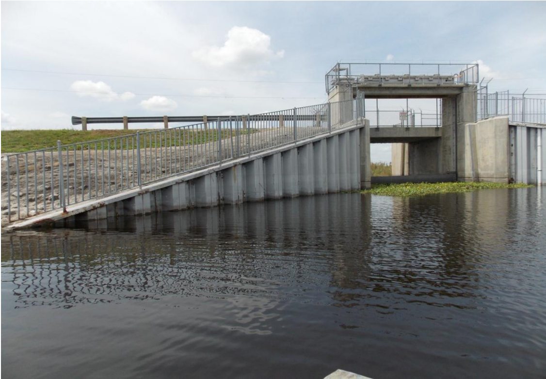
Upstream - South Wing Wall and Structure.
