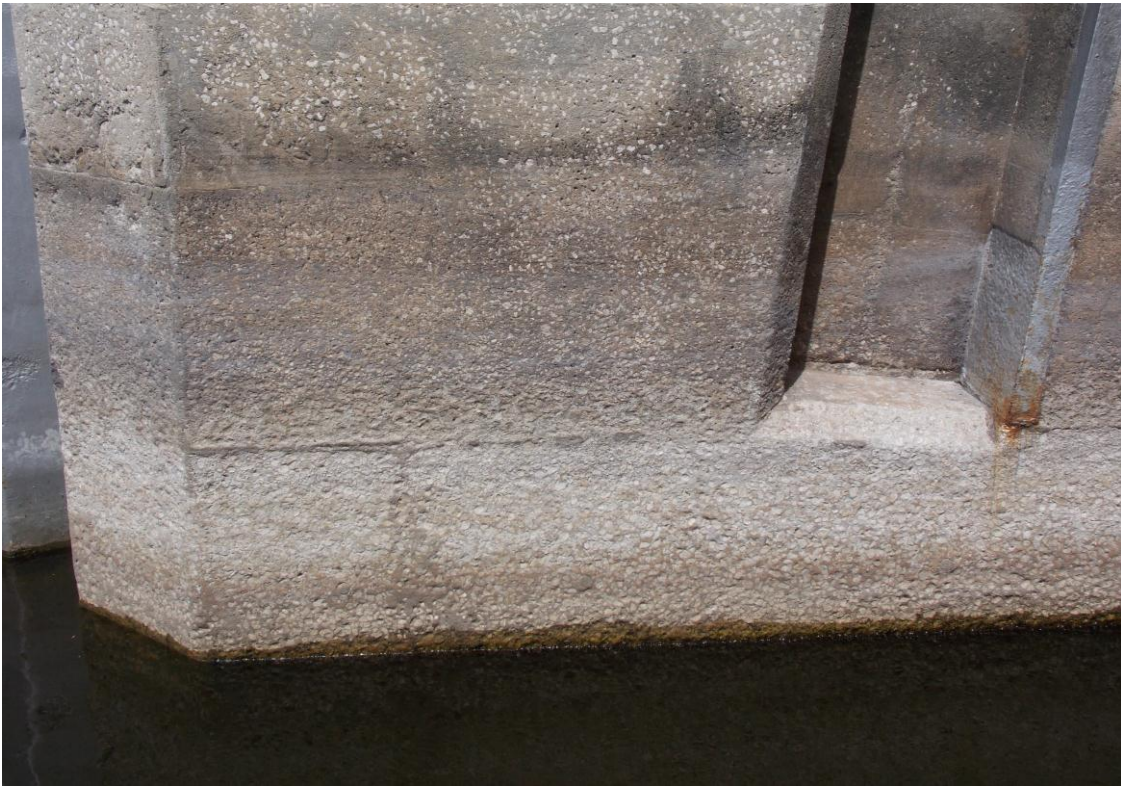
Downstream -South Structure Wall.
