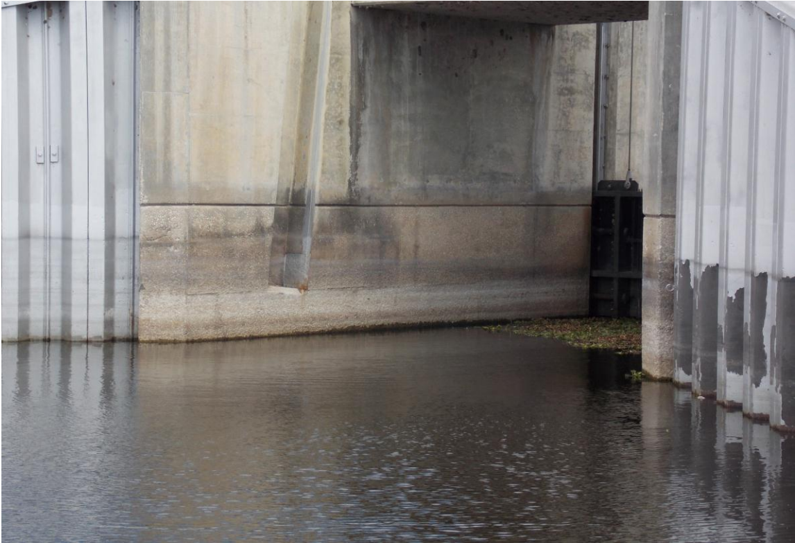
Downstream - North Structure Wall.
