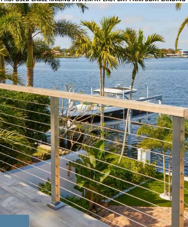
PROPOSED CABLE RAILING SYSTEM AT EAST BAY PARK BOAT LANDING
