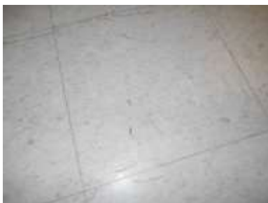
HOMOGENEOUS AREAS 12, 13 12" FLOOR TILE (BEIGE)/MASTIC
