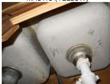
HOMOGENEOUS AREA 14 SINK COATING
