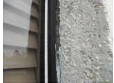
HOMOGENEOUS AREA 18 EXTERIOR CAULK
