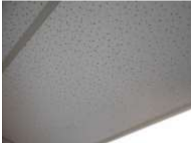
HOMOGENEOUS AREA 01 2' X 4' CEILING TILE
