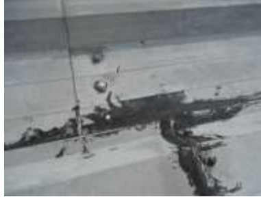
HOMOGENEOUS AREA 17 METAL ROOF TAR
