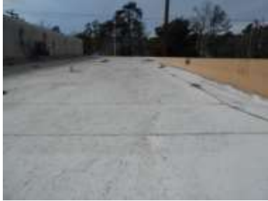
HOMOGENEOUS AREA 16 EPDM ROOF MEMBRANE
