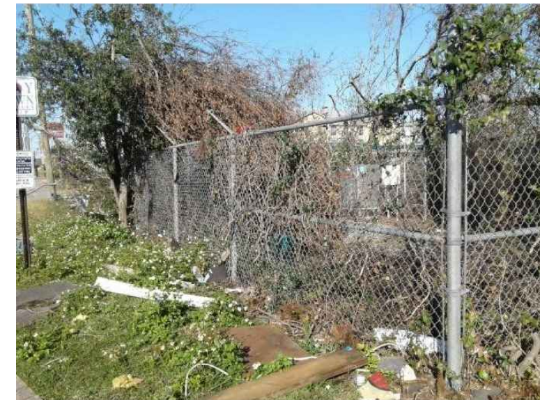
INSTALLATION OF LIFT STATION FENCE REPAIR
