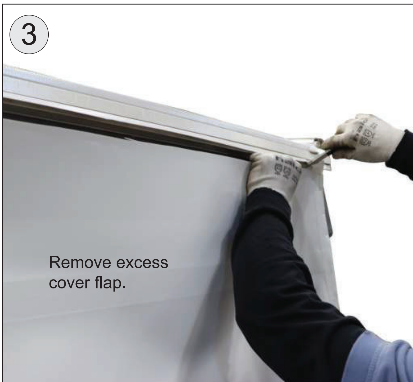
3. Once poly lock is seated, carefully trim excess cover material.
