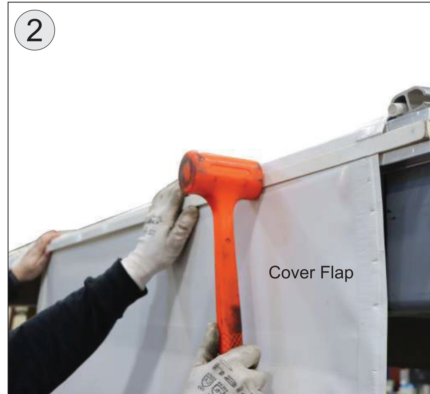
2. Using a dead-blow mallet, set poly lock strip in channel to lock cover.
