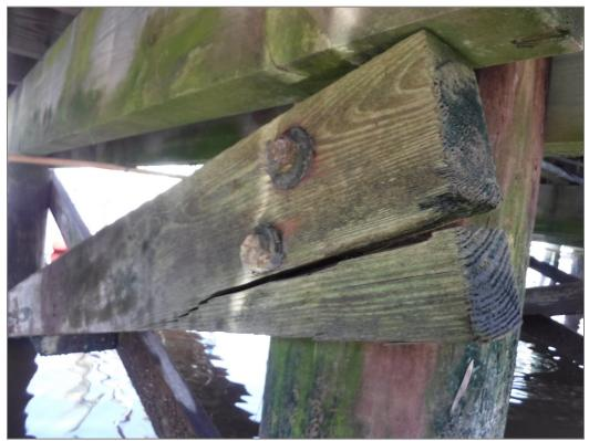
Photo 16: Cross Brace – Split at end with heavily corroded hardware (Major, Sta. 4+95)
