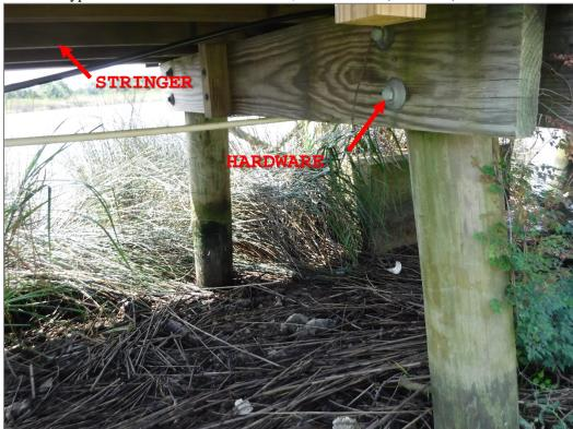
Photo 2: Typical Bent – Northwestern section, 8 foot wide (Sta. 13+70)
