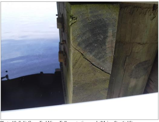
Photo 18: Split Cap – End View, Full penetration crack (Major, Sta. 6+15)
