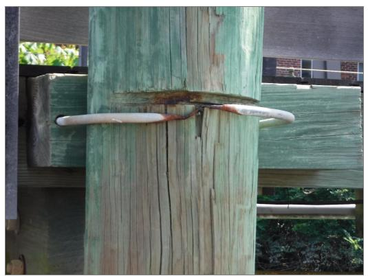
Photo 10: Fender Pile Hardware – Severe Condition (Failed, Sta. 0+49)
