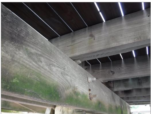
Photo 5: Underside – Typical condition stringer and pile cap
