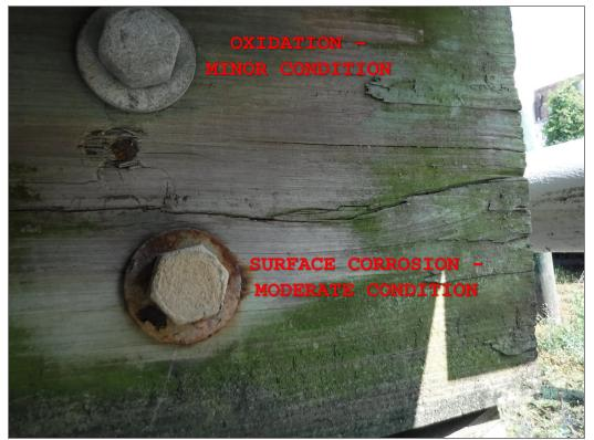
Photo 8: Hardware – Typ. surface corrosion (bottom) and oxidation of galvanization (top)
