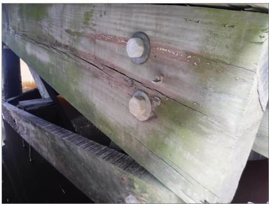
Photo 17: Split Cap – Face View, Full penetration crack (Major, Sta. 6+15)
