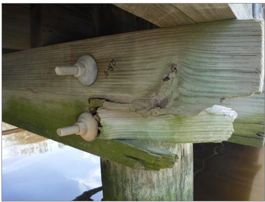
Photo 21: Split Cap – Impact damage on outboard end (Major, Sta. 10+80)
