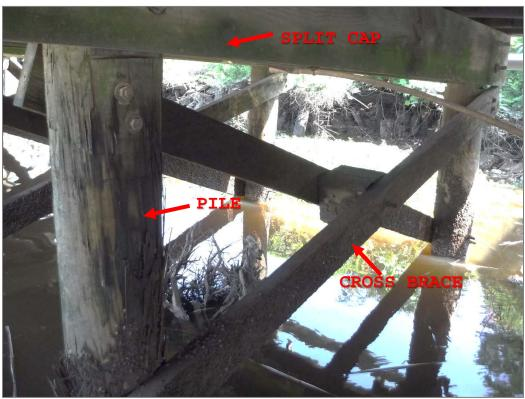
Photo 1: Typical Bent – Southeastern section, 12 foot wide (Sta. 0+30)
