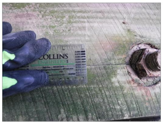
Photo 4: Split Cap – Typical minor crack, typical fungal growth (Minor, Sta. 0+30)
