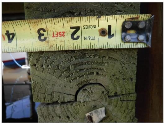
Photo 14: Split Cap – End View, Full penetration crack (Major, Sta. 2+60)
