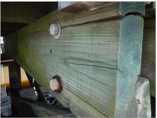
Photo 20: Split Cap – Full penetration crack (Major, Sta. 8+15)
