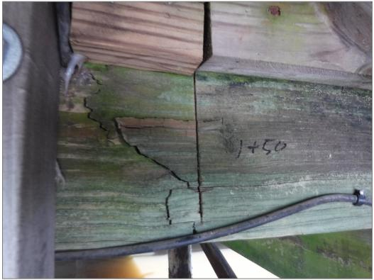
Photo 6: Stringer – Cracking on fascia (Minor, Sta. 1+50)
