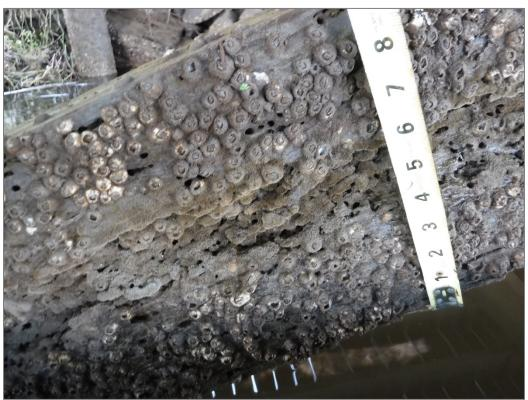
Photo 11: Cross Brace – Major marine borer damage (Major, Sta. 0+10)
