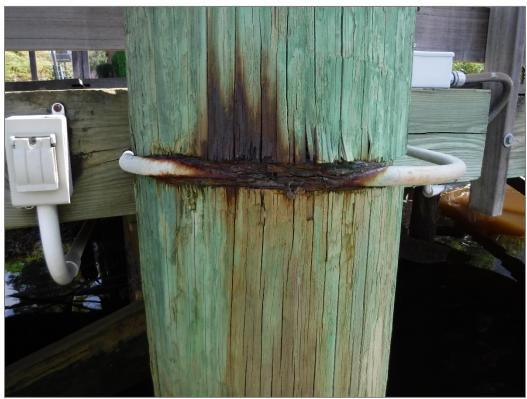
Photo 9: Fender Pile Hardware – Severe Condition
