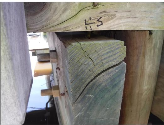
Photo 19: Split Cap – Full penetration crack (Major, Sta. 7+65)
