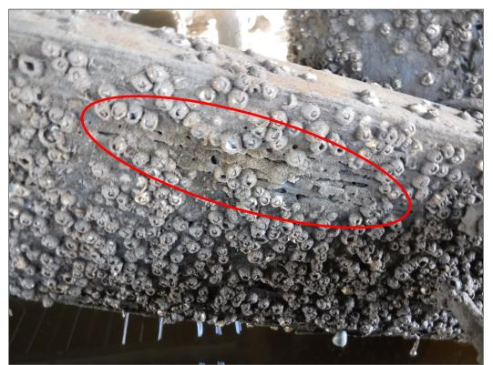
Photo 12: Cross Brace – Typical marine borer damage (Moderate, Sta. 0+15)
