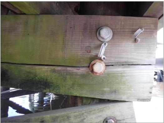
Photo 13: Split Cap – Face View, Full penetration crack (Major, Sta. 2+60)
