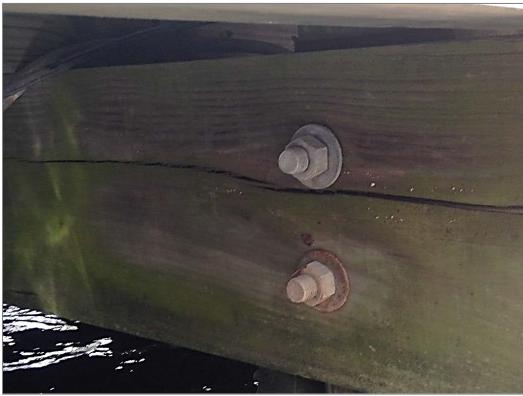
Photo 15: Split Cap – End View, Full penetration crack (Major, Sta. 2+90)
