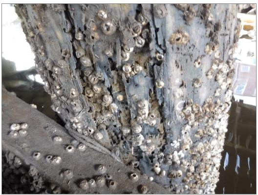
Photo 3: Pile – Typical marine borer damage (Moderate, Sta. 0+10)
