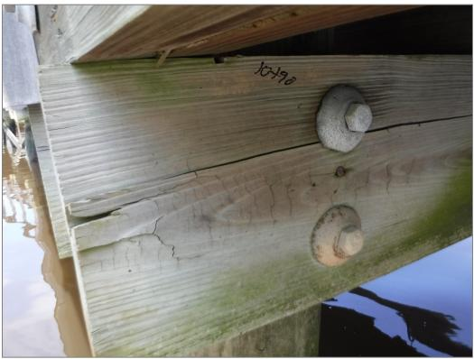
Photo 22: Split Cap – Full penetration crack (Major, Sta. 10+90)
