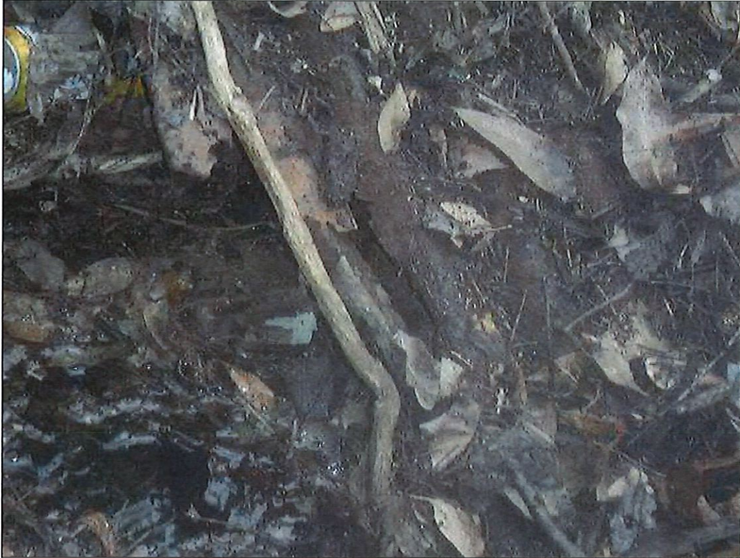
SECTION LOSS LINE 4 FROM SOUTH END BACK 1.0'(PAR)
