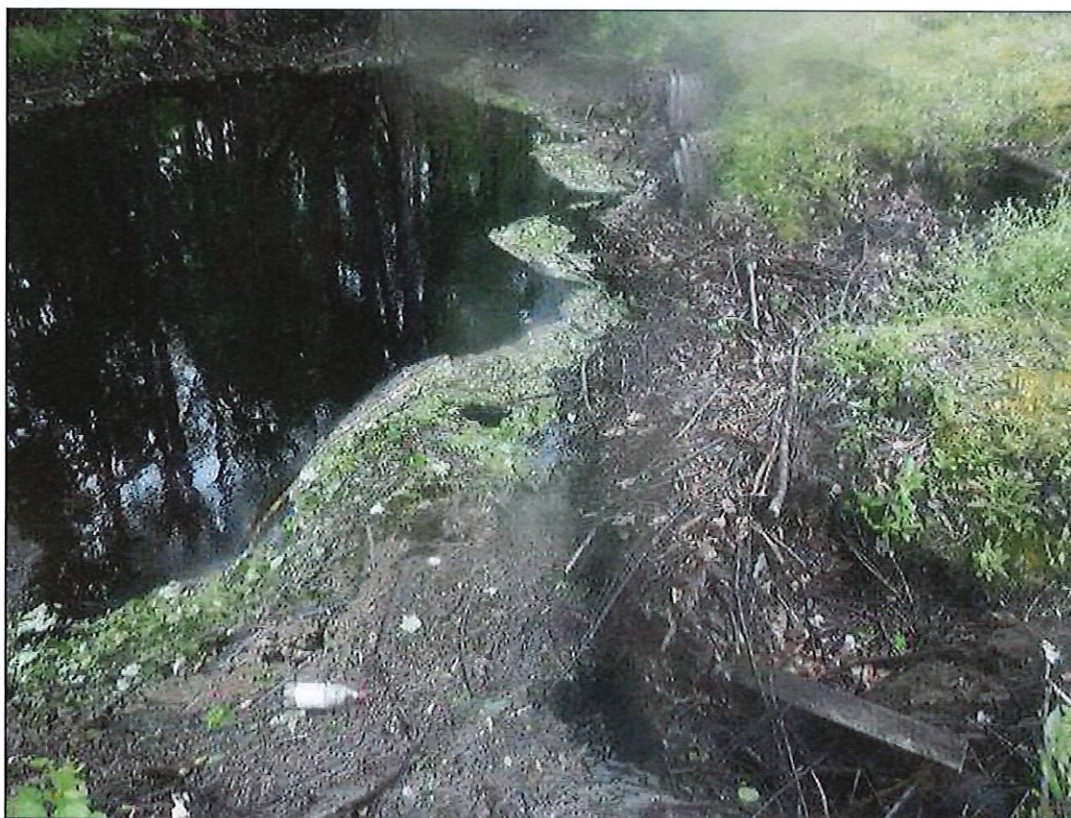
DRIFT FROM MUDLINE TO 1' ABOVE TOP OF ALL LINES AT THE SOUTH END EXTENDING INTO PIPES +/- 5.0' (PAR)
