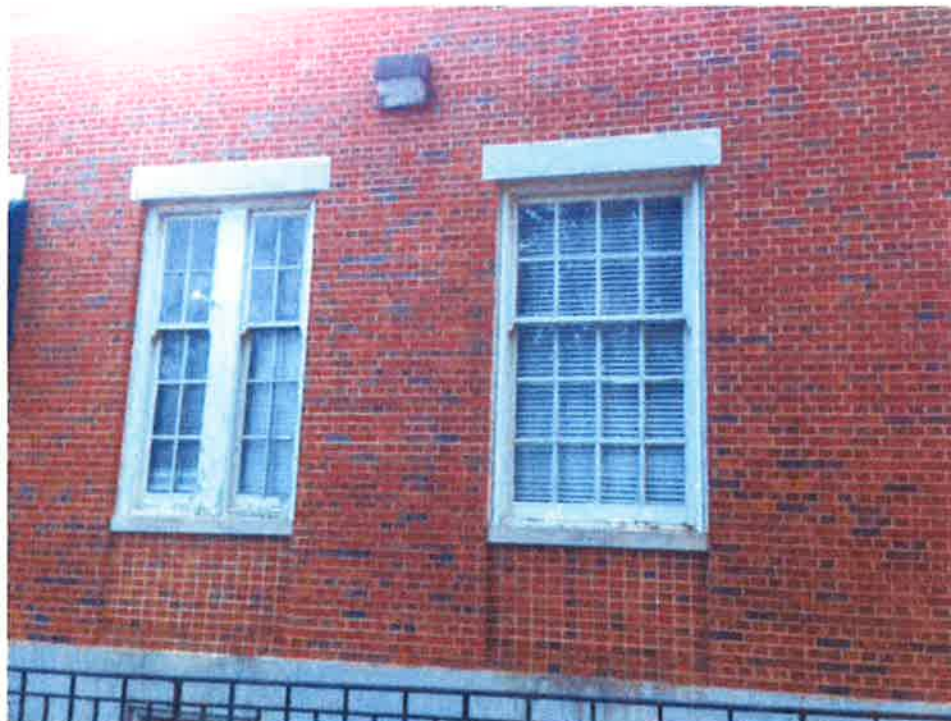
Photo 22: Typical Type J & K Window Configuration - Exterior
