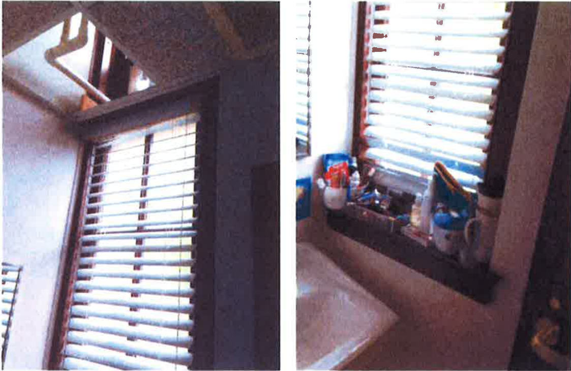
Photo 23: Typical Type K & L Window Configuration - Interior
