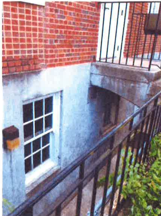
Photo 26: Typical Type O Window Configuration - Exterior
