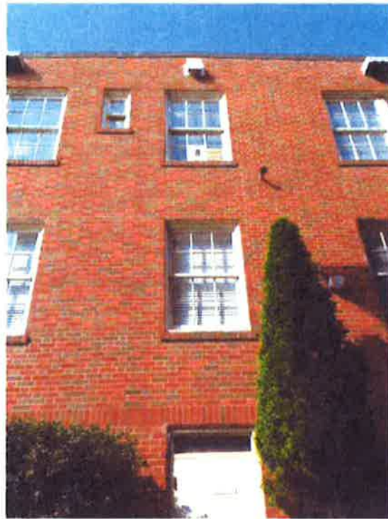
Photo 21: Typical Type A & B Window Configuration – Exterior
