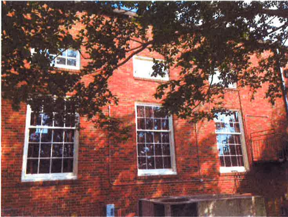
Photo 19: Typical Court Room Type C & D Window Configurations - Exterior
