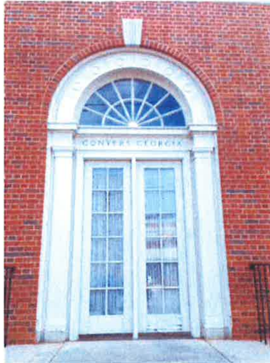
Photo 28: Type P Window & Type 1 Door Configuration - Exterior
