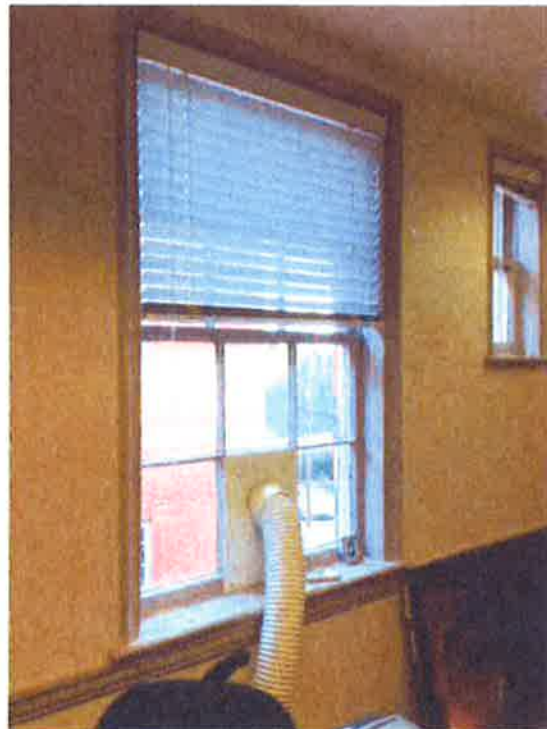
Photo 18: Typical Type A & B DH Window Configuration - Interior
