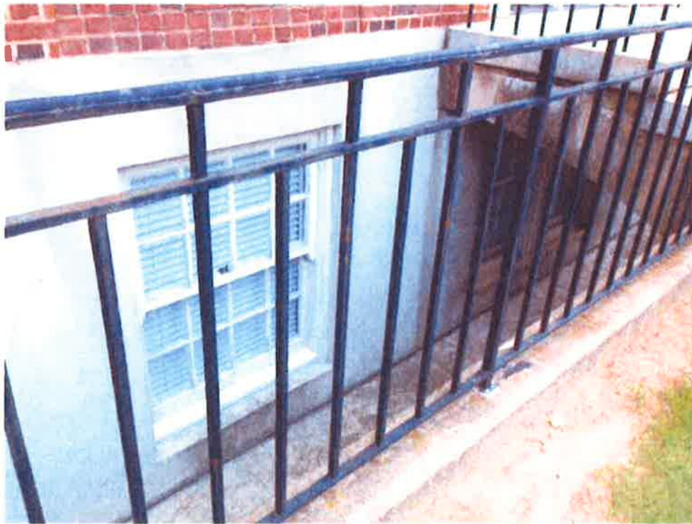
Photo 24: Typical Type M & N Window Configuration - Exterior
