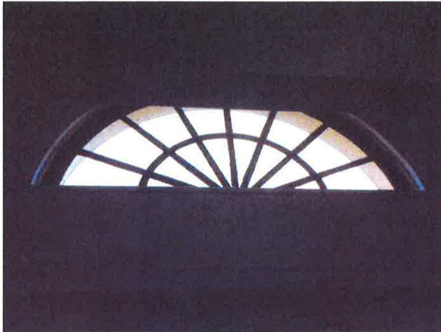
Photo 29: Window Type P Configuration - Interior
