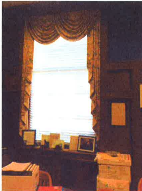
Photo 15: Typical Type C, J & D Sim. Window Configuration – Interior
