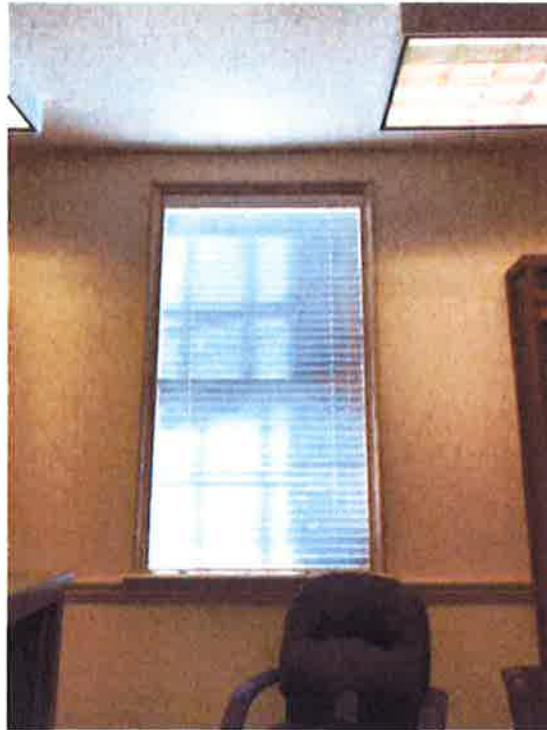
Photo 17: Typical Type F, H & I DH Window Configuration - Interior
