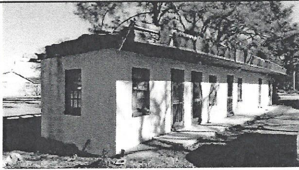
Picture 3 – Rear of Building
