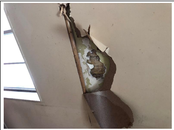
11. 1385 32nd St., Apts A & B - White Textured Material w/ Paint (Unit B Bedroom): HSA 21.
