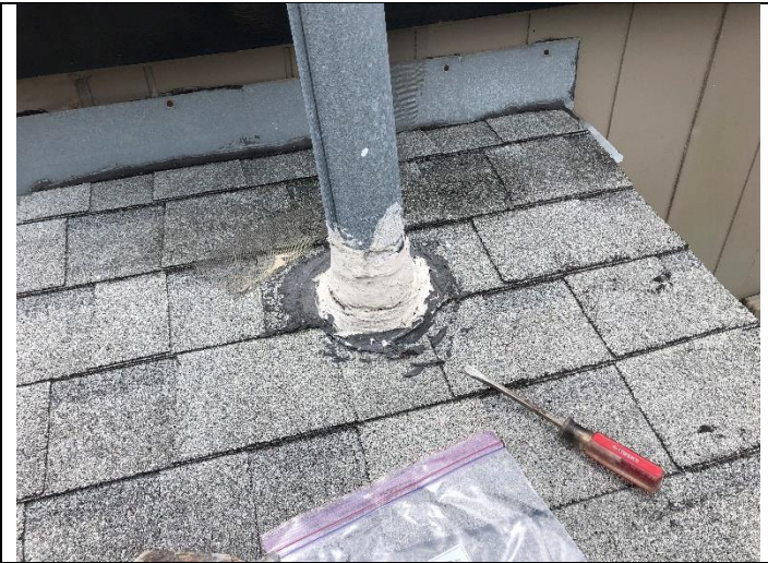
15. 3136-3146 US 1 - Black Roof Flashing & Silver Coating Material (Roof Stacks): HSA 33.
