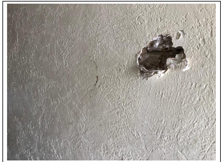
12. 1385 32nd St., Apts A & B - Rough Textured Wallboard Ceiling (Unit B Bedroom): HSA 22.
