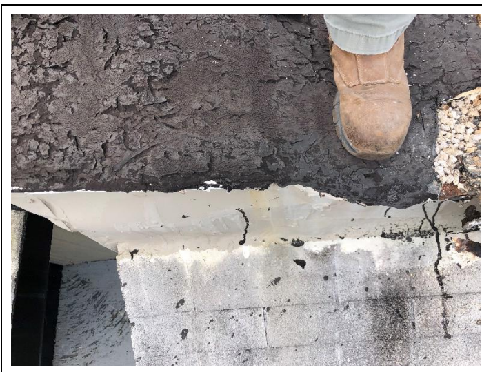
6. 1385 32nd St., Apts A & B - Black Tar (Roof Seams Under Eaves): HSA 4.
