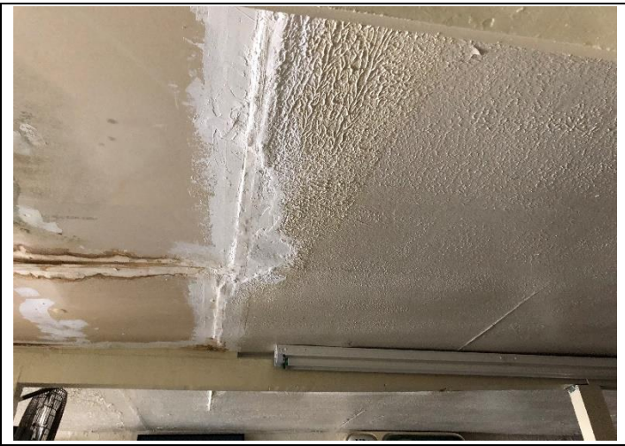
19. 3136-3146 US 1 - White Textured Material w/ Paint (Main Room Walls & Ceiling): HSA 41.
