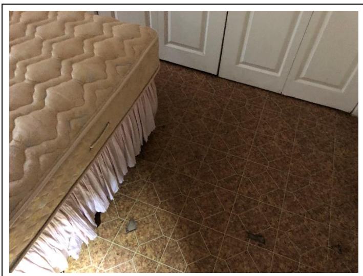
3. 1375 32nd St - Gray Vinyl Floor Tile & Black Mastic (Unit A Bathroom & Bedroom Doorways): HSA 22.
