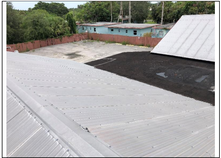
14. 3136-3146 US 1 - Silver Coating Material (Btwn Metal Roof Pitch): HSA 30.
