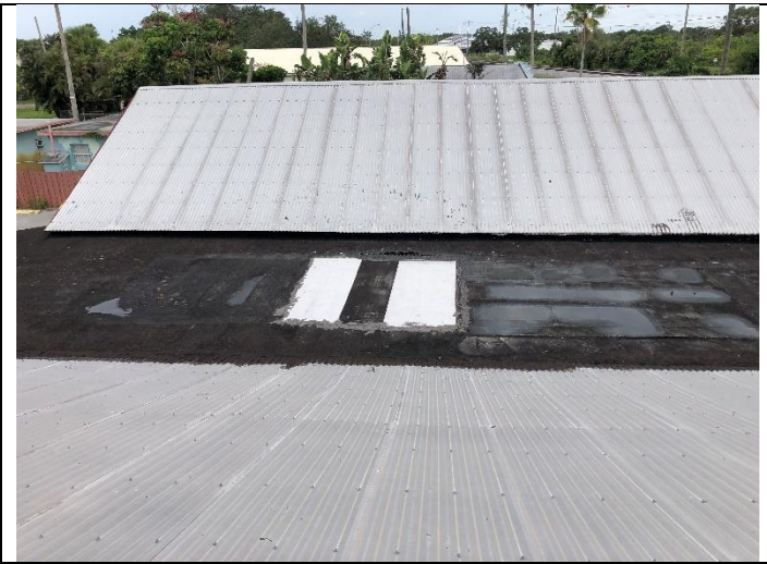
13. 3136-3146 US 1 - Silver Coating Material (Btwn Metal Roof Pitch): HSA 29.
