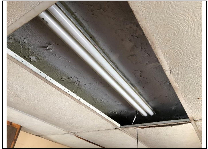
10. 1385 32nd St., Apts A & B - White Surfacing Material w/ Paint (Unit A Kitchen, Living Room & Bathroom): HSA 19.
