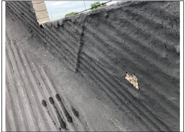
16. 3136-3146 US 1 - Black Tar & Silver Coating Material (Parapet Front of Bldg.): HSA 36.
