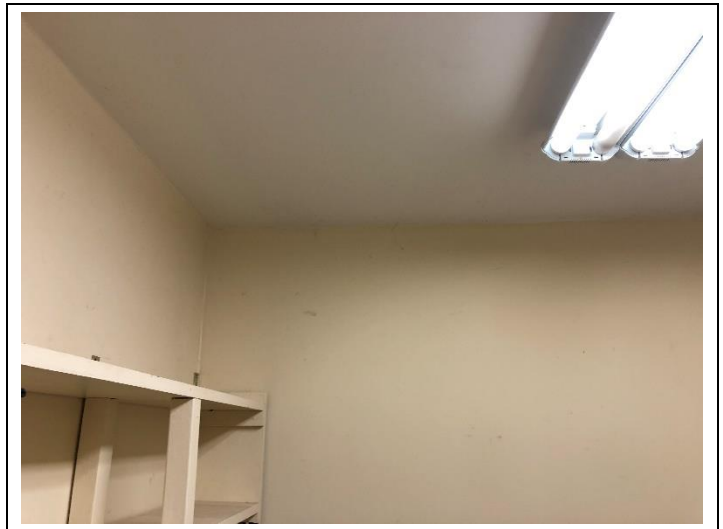
18. 3136-3146 US 1 - White Surfacing Material w/ Paint (Bldg. Interior): HSA 38.
