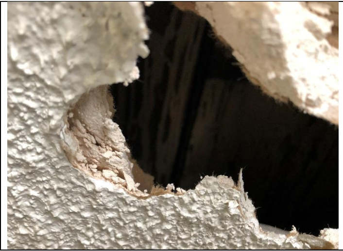
9. 1385 32nd St., Apts A & B - White Textured Material w/ Paint (Unit A Bedroom): HSA 14.
