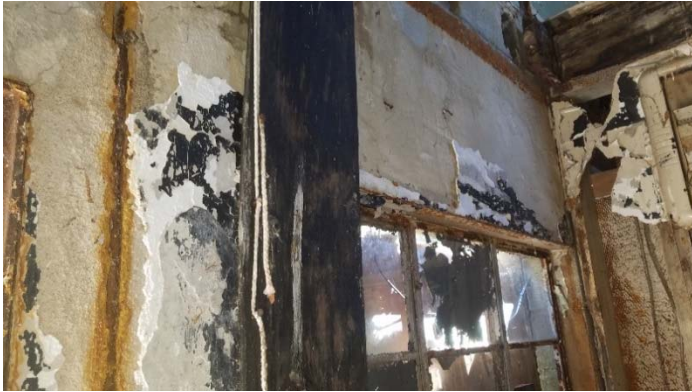
Photo 7 – Plaster over dry wall.
