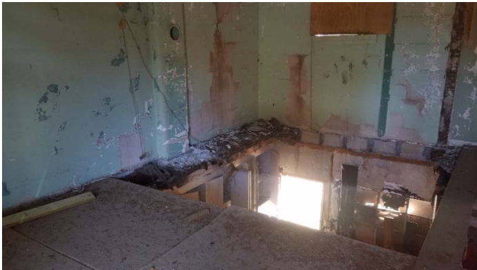
Photo 9 – 1 st floor plaster over drywall.
