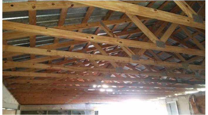
Photo 2 – New metal and wood roof system.
