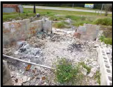
11: Partial Block Structure (#8).
