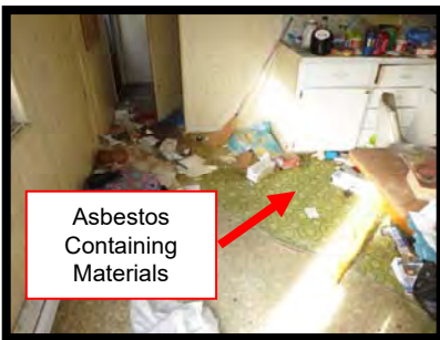
3: View of green linoleum in kitchen area.
