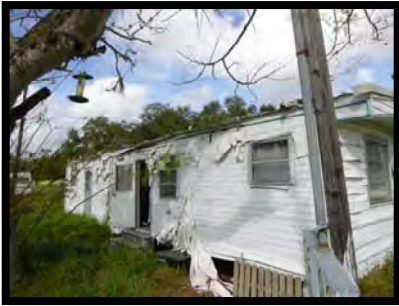
3: Trailer Unit C.
