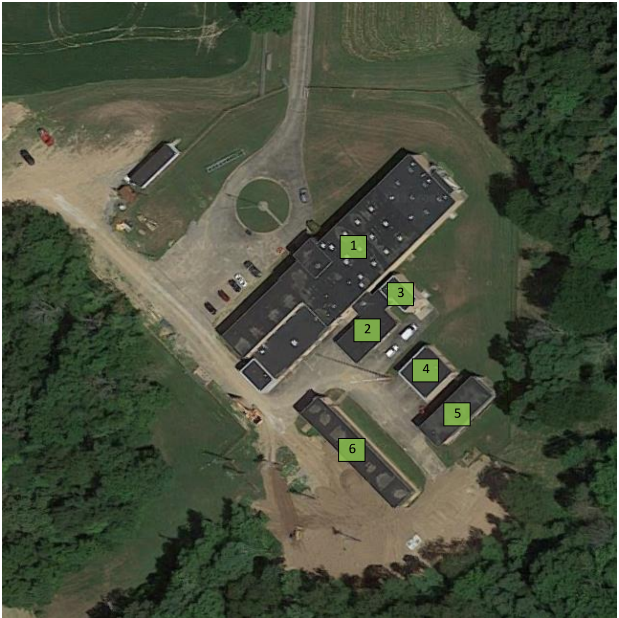
Figure 3.18 Sugar Creek WTP Facilities
