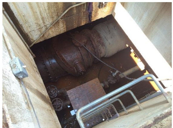
Figure 3.28 Surge Tank Valve Vault
