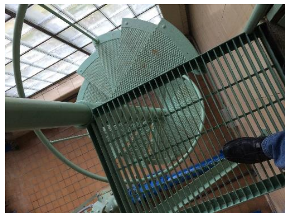
Figure 3.24 HS Pump Room Stairs to 2 nd Floor Control Room
