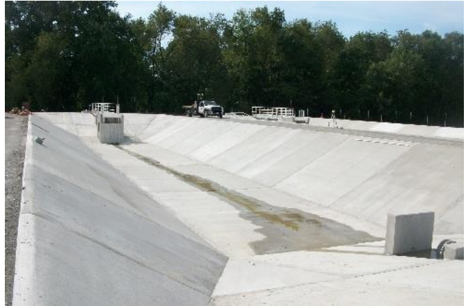
Figure 3.9 Backwash Lagoons Filters
