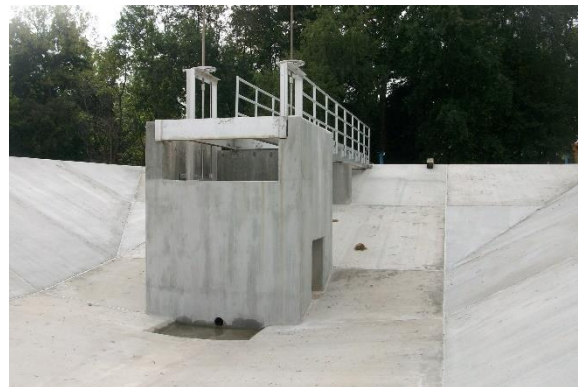
Figure 3.13 Backwash Lagoon Overflow Control Structure
