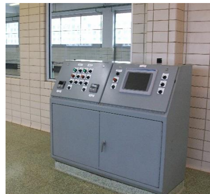
Figure 3.8 Filter Consoles
