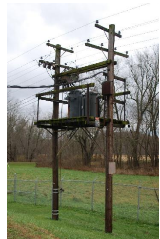
Figure 3.3 Electrical Feed to Wells
