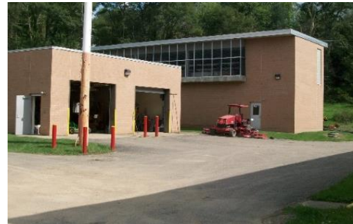
Figure 3.23 Maintenance Building (East Aerator in Background)
