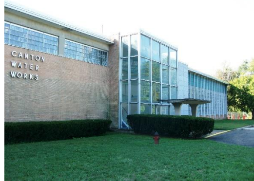
Figure 3.19 Front of WTP Main Building
