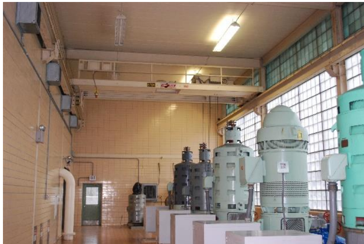
Figure 3.15 High Service Pump Room
