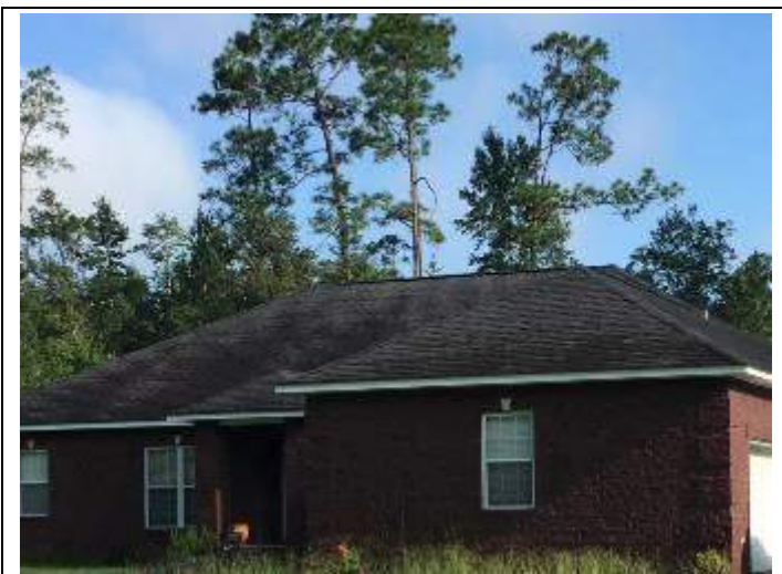
5. View of HSA-5 and HSA-6: Black Asphalt Roof Shingles, Felt, and Mastic.
