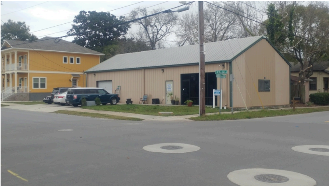
Photo 20: VIEW OF NORTH ADJOINING PROPERTIES.
