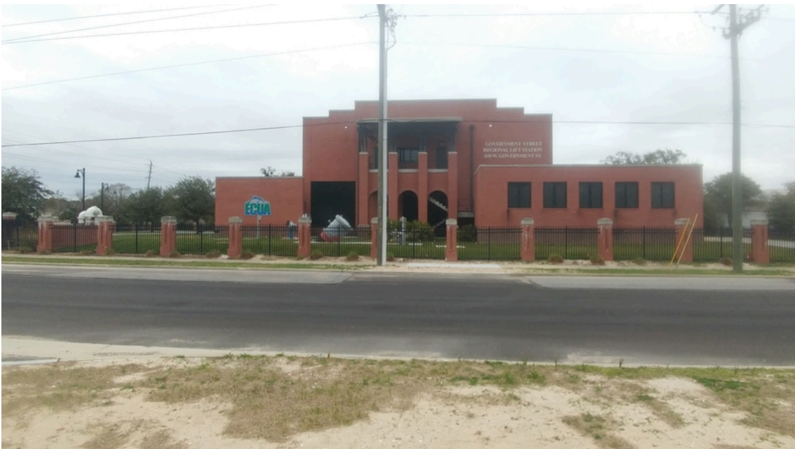
Photo 24: VIEW OF NORTH ADJOINING PROPERTIES.
