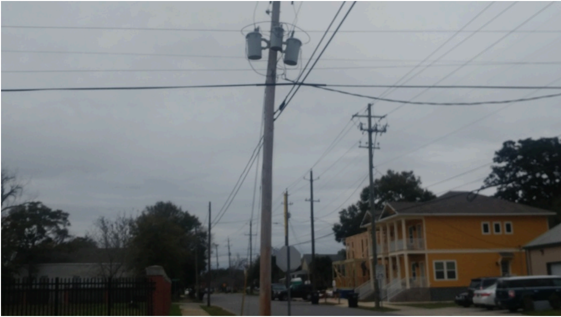
Photo 23: VIEW OF NORTH ADJOINING PROPERTY, POLE-MOUNTED TRANSFORMER.
