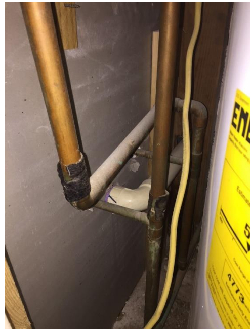
8. Representative view of pipe insulation material (SV5-19 - SV5-21)
