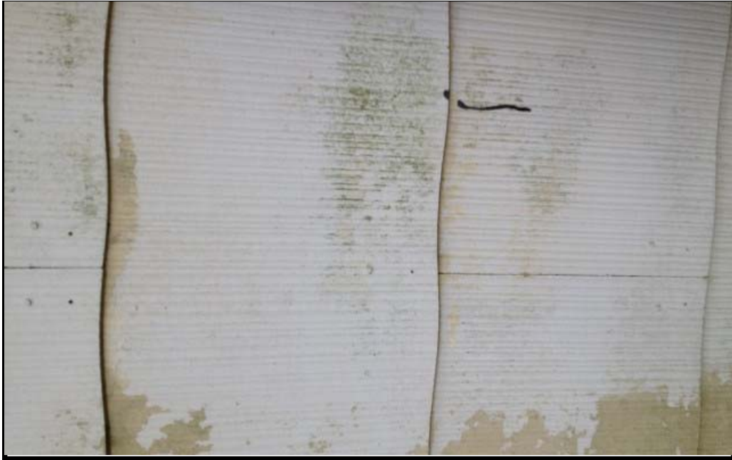
Photo 5: Cement Board Exterior Siding.
