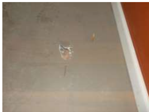
HOMOGENEOUS AREAS 06, 07 VINYL SHEET FLOORING (WOOD) MASTIC (BEIGE)
