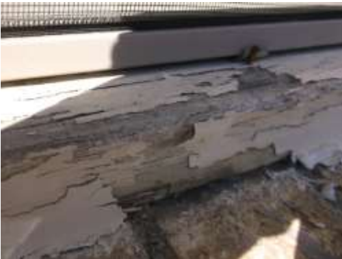
HOMOGENEOUS AREA 11 WINDOW/DOOR CAULK
