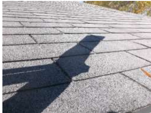
HOMOGENEOUS AREA 12 ROOF SHINGLE
