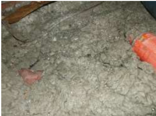
HOMOGENEOUS AREA 03 ATTIC INSULATION
