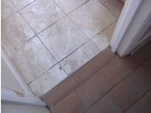
HOMOGENEOUS AREA 01 CERAMIC TILE GROUT
