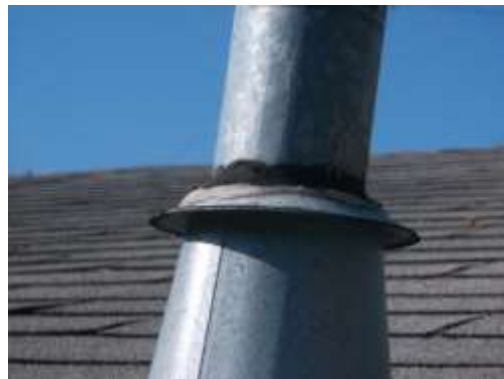
HOMOGENEOUS AREA 14 ROOF CEMENT (BLACK)
