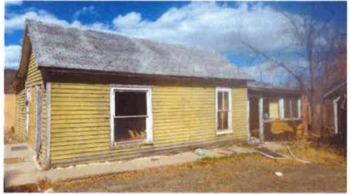
Structure 1 – Framed House
