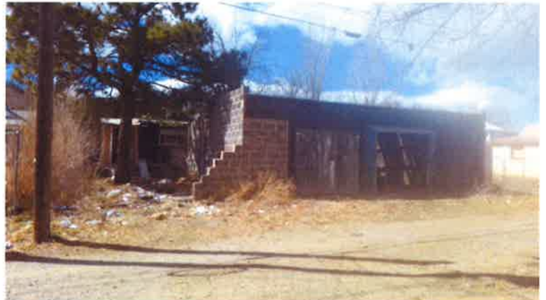
Structure 3 – Cinder Block Garage From Alley
