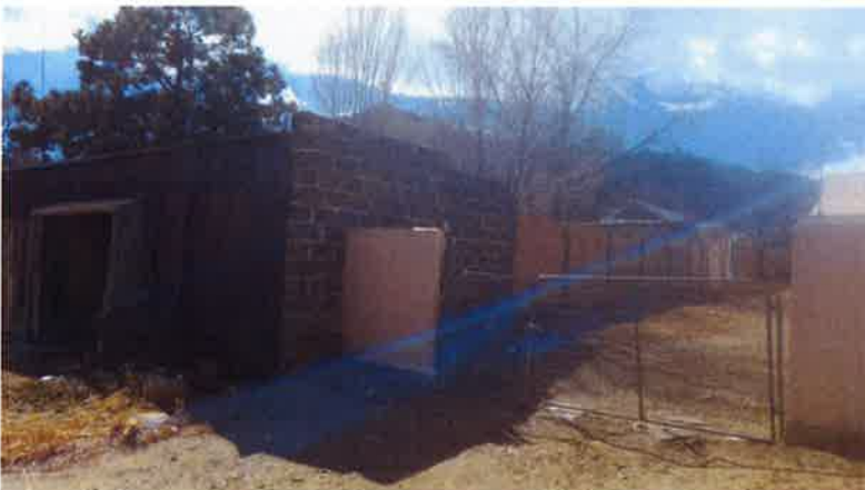
Structure 3 – Cinder Block Garage
