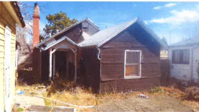
Structure 2 – Framed House
