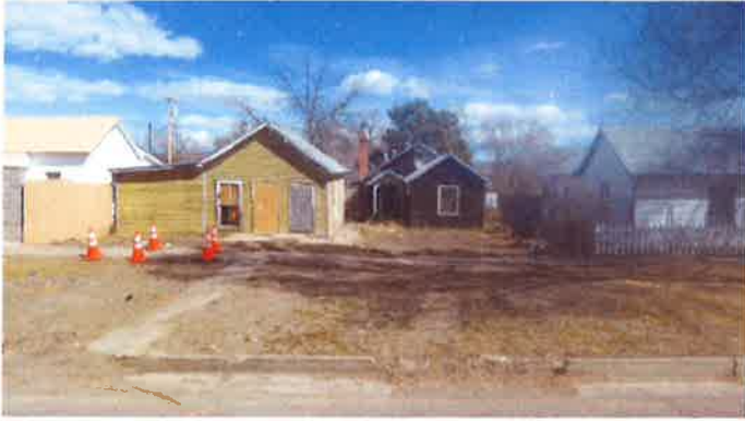
Structure 1 and Structure 2 From Street
