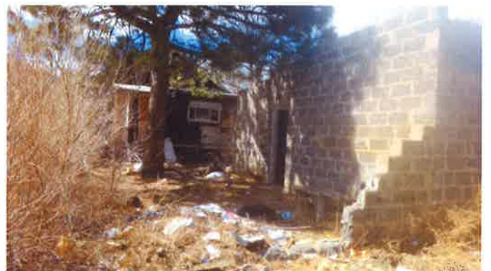
Structure 3 – Cinder Block Garage
