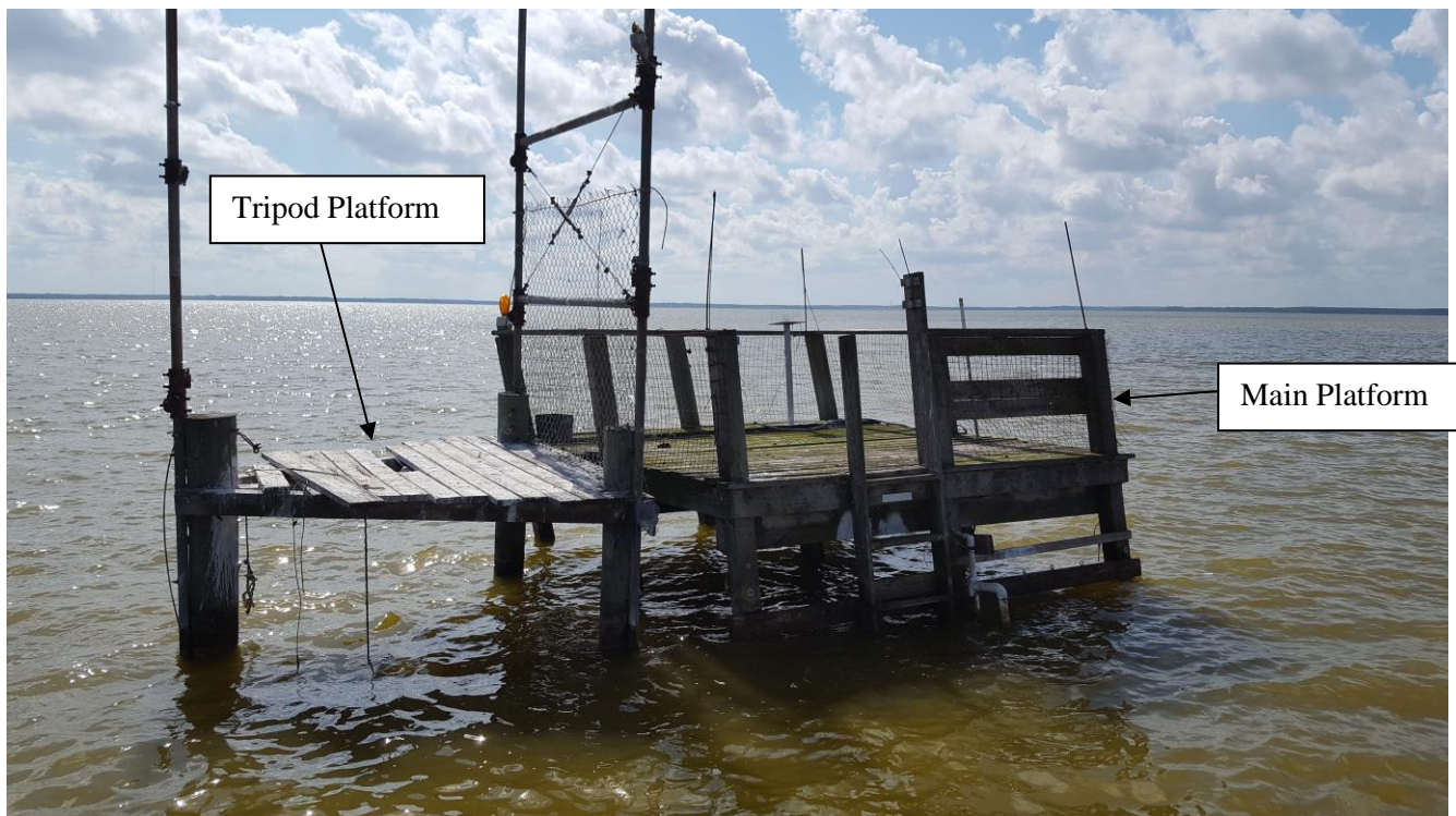
Dimensions of structures: main platform: 12ft. x 12 ft. (right side of photo), Tripod Platform: 10ft. each side (left side of photo)
