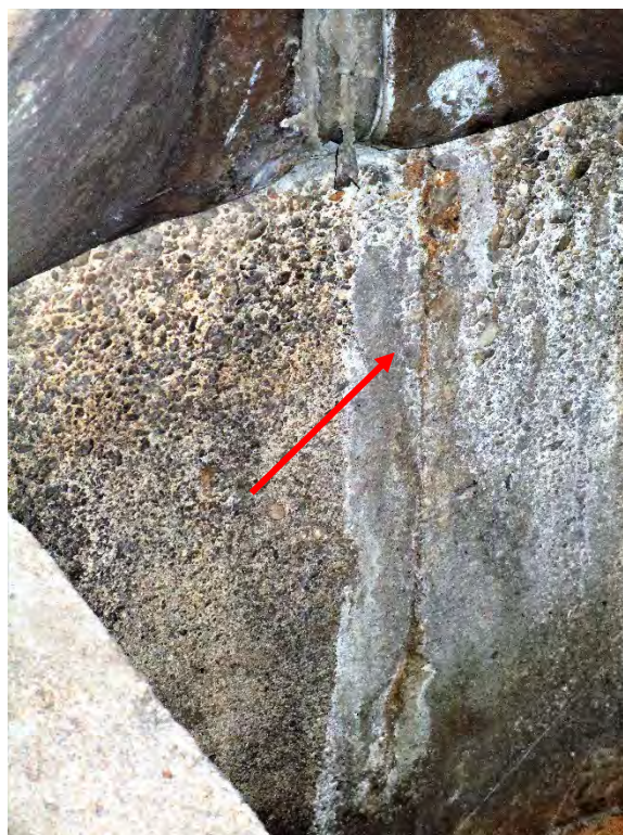
Photo A-4. Launder Joint
