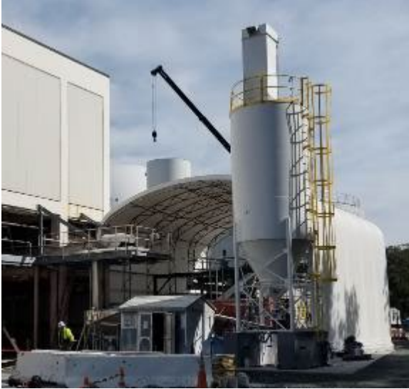
Figure 22-3. Temporary Lime Stabilization in Howard County, Maryland
