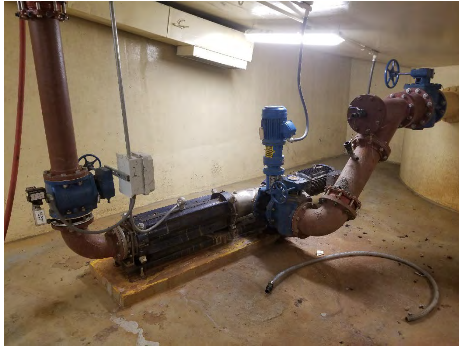
Figure 8. Gravity Thickener Pump
