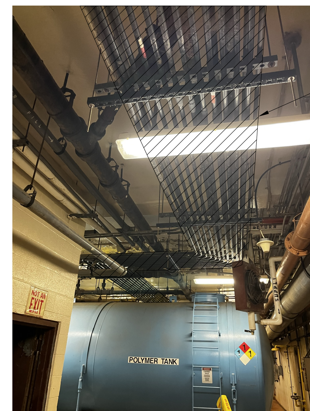
5 DWB TUNNEL-CEILING M-002
