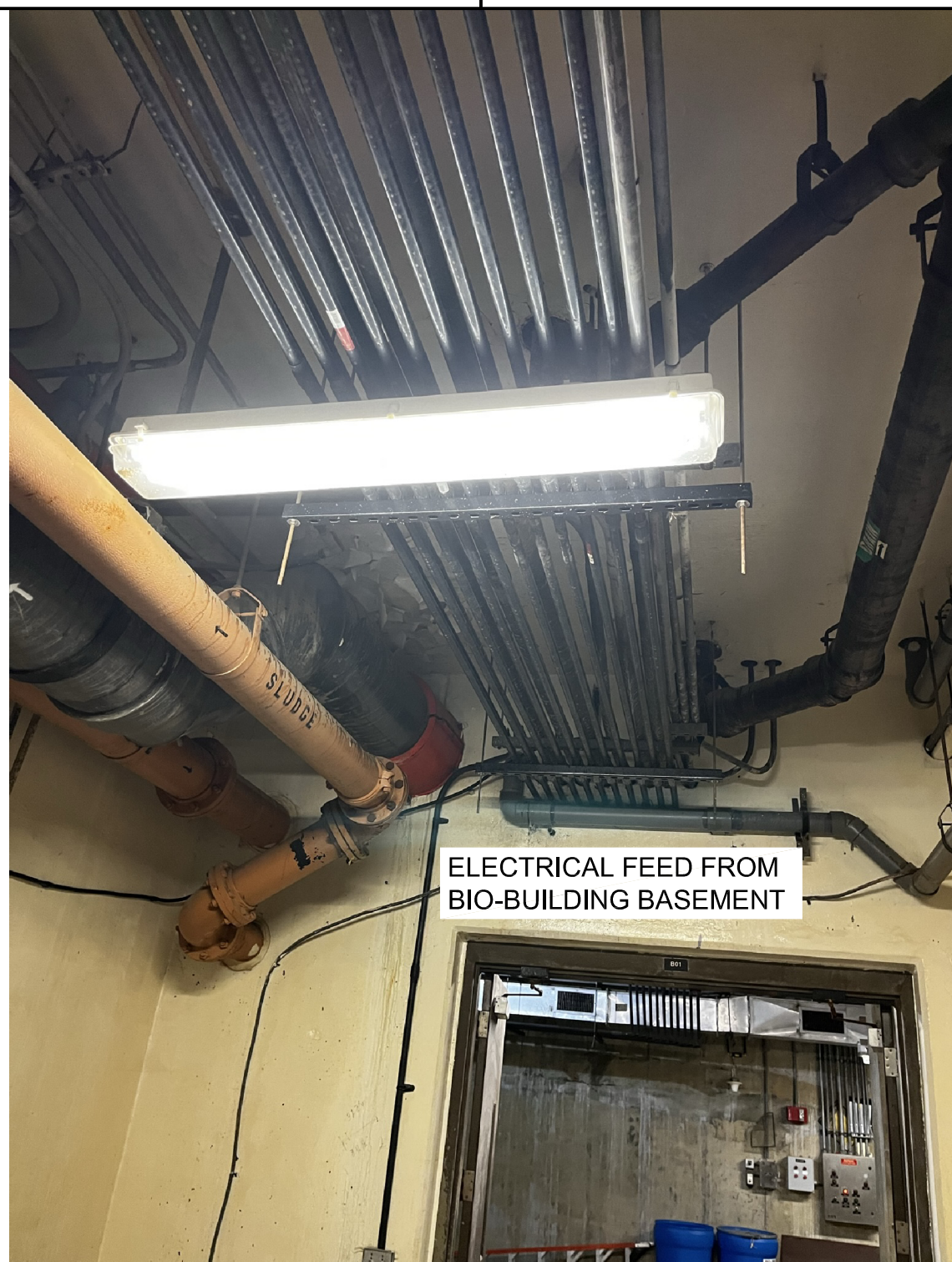
6 BIO-BUILDING LOOKING TOWARD DWB TUNNEL M-002
