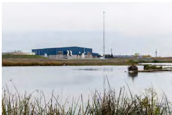
Image from Stantec website 1/14/2022: www.stantec.com/en/projects/canada-projects/g/grand-bend-area-wwt-facility
