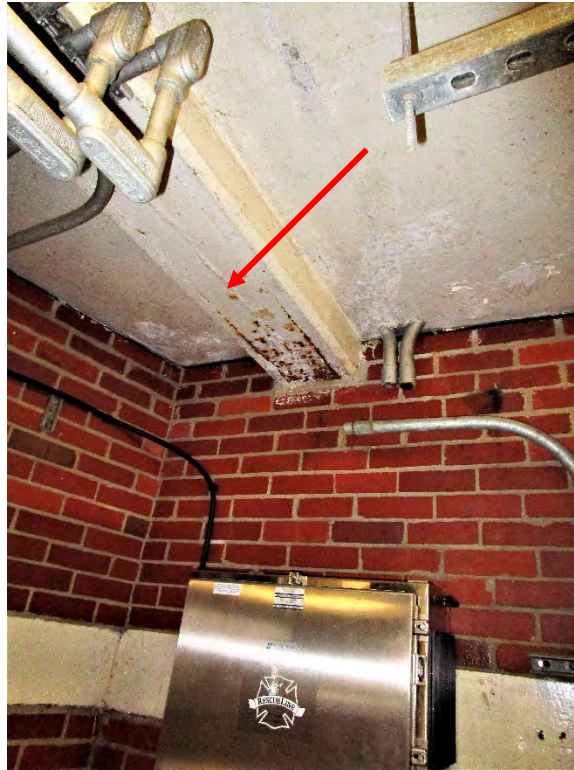
Photo A-23. PS Roof Beam
