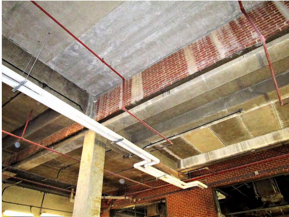
Photo A-37. Extension to Loadout
