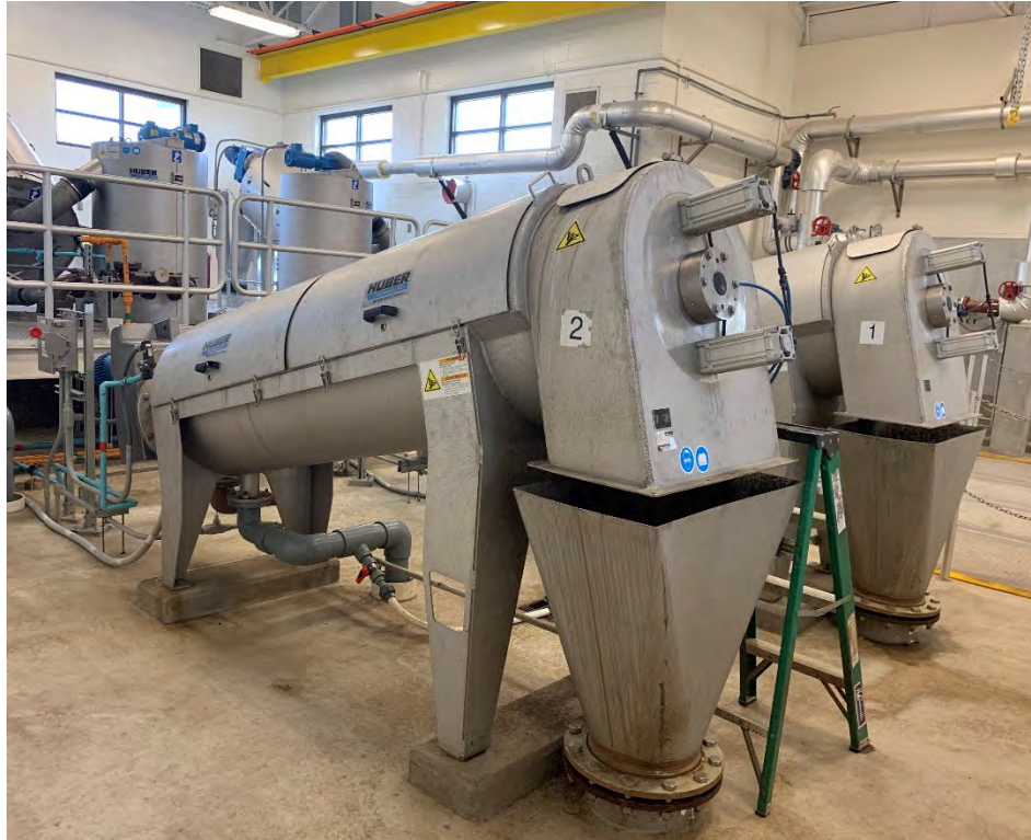
Figure 7. Screw Press
