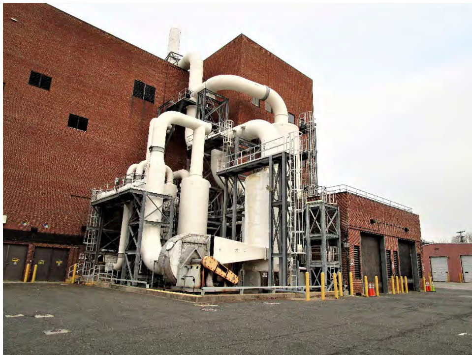
Photo A-27. Dewatering Building from East
