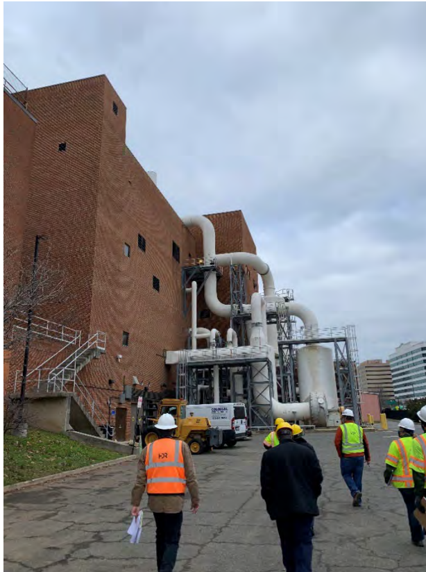
Figure 15. Area Where Fan outside the Dewatering Building Is Located
