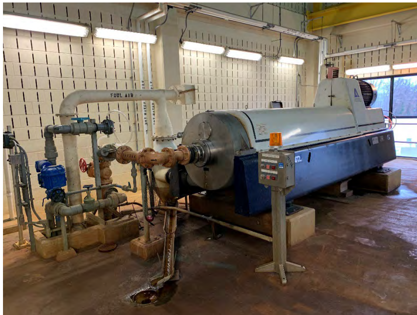
Figure 13. Dewatering Centrifuge
