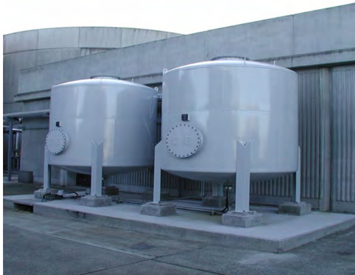
Figure 1. Adsorptive Media Installation Example
