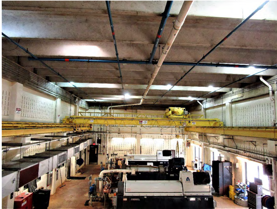
Photo A-41. Centrifuge Room and Double Tee Roof
