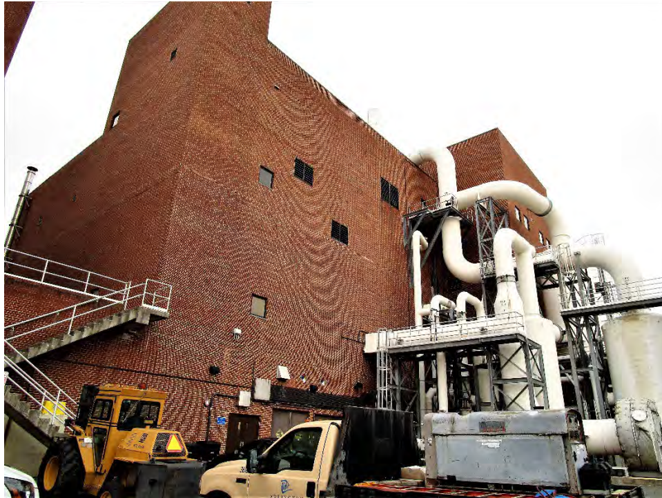
Photo A-26. Dewatering Building from Southeast
