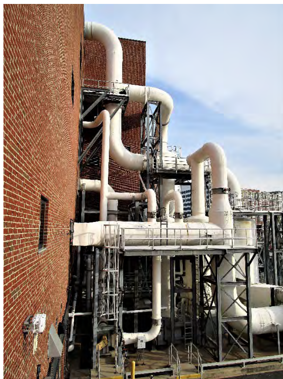
Photo A-48. Odor Control System To Be Demolished
