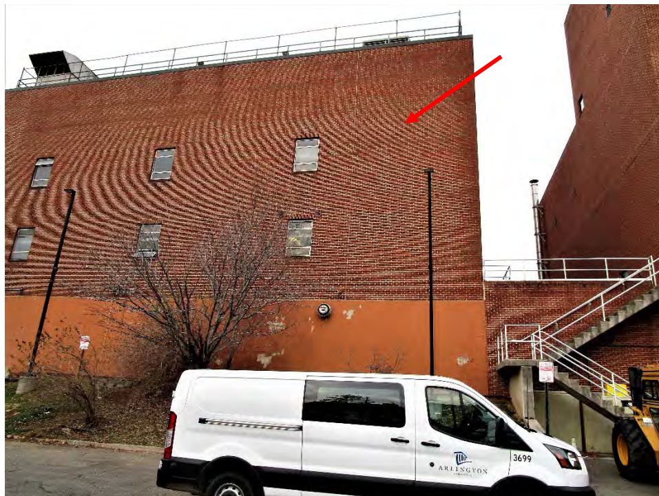
Photo A-28. Bio-Building to Demolish (Photo 1 of 2)
