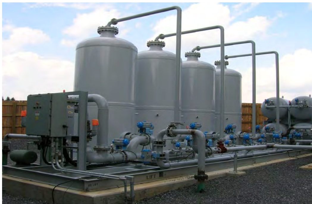
Figure 13. Typical PSA Installation
