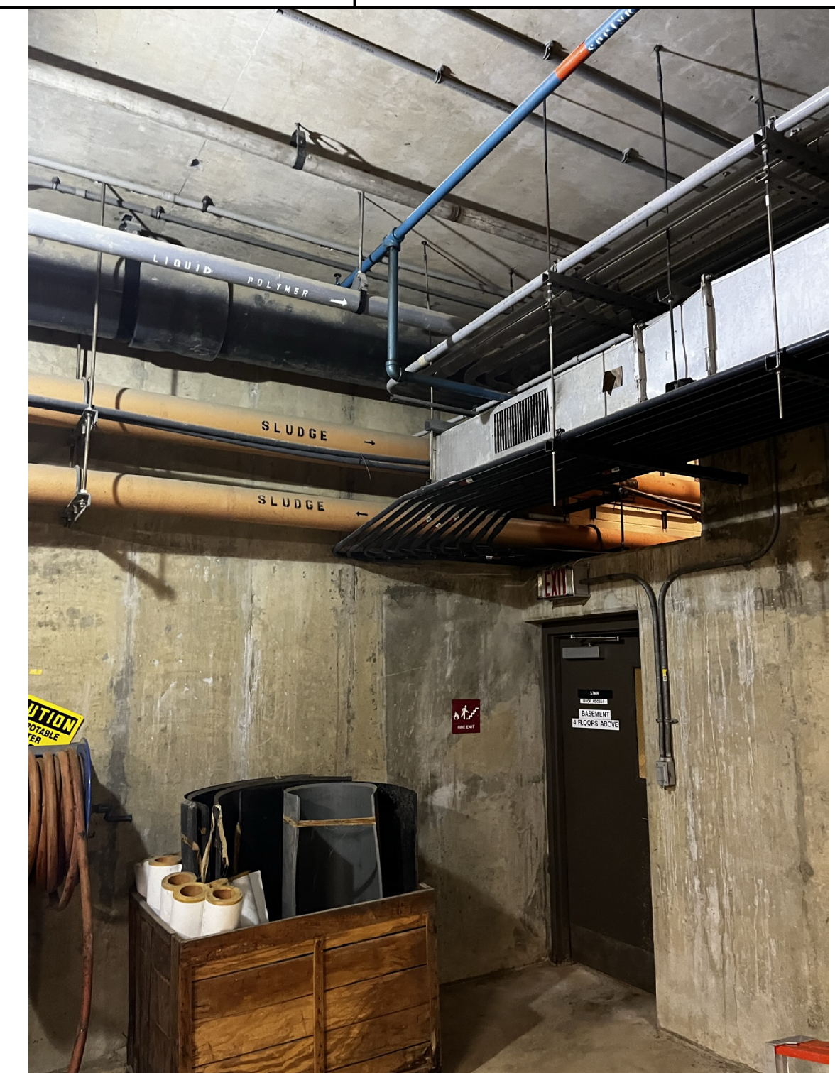
8 DWB TUNNEL-NORTHWEST CORNER M-002
