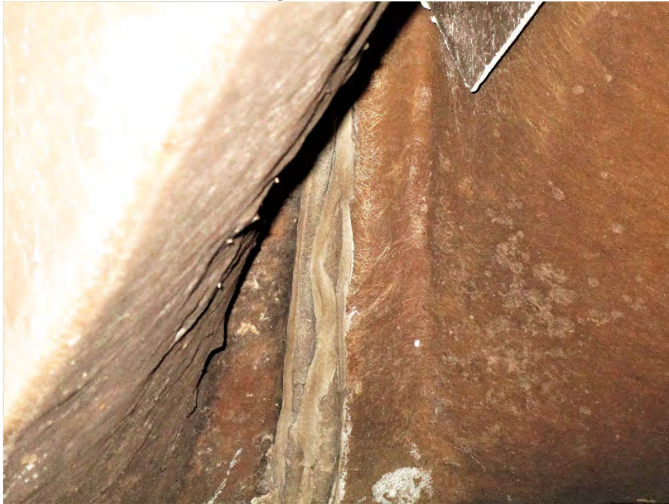
Photo A-14. FRP Joint
