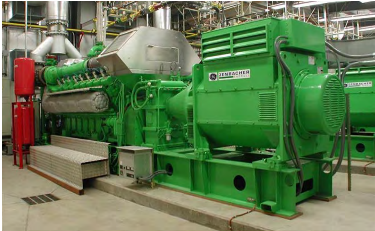
Figure 11: Typical Engine Installation
