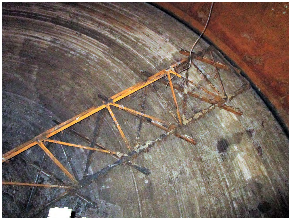
Photo A-1. Mechanical Scraper—To Be Replaced
