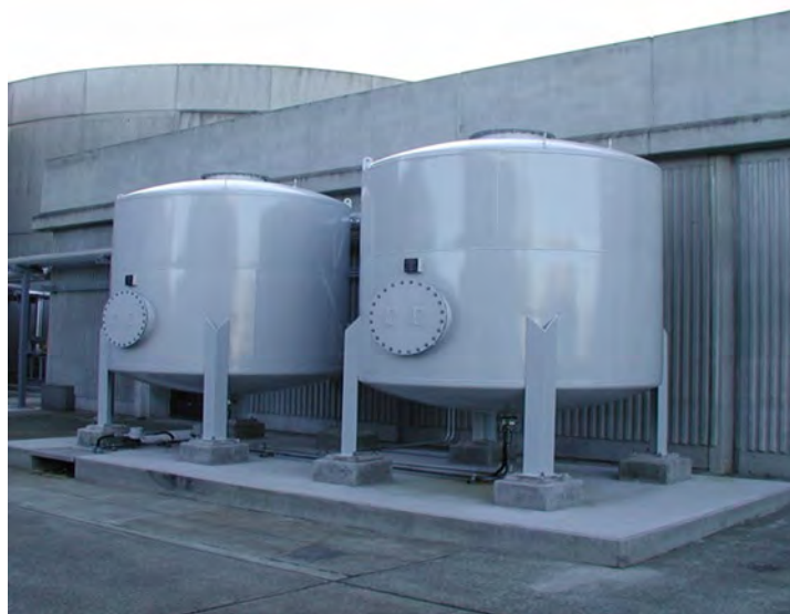
Figure 1. Adsorptive Media Installation Example
