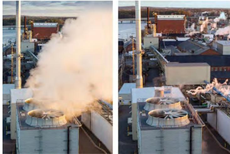
Figure 9. Evaporative Cooling Tower Example: Left Side Operating with Plume Abatement Off, Right Side Operating with Plume Abatement On
