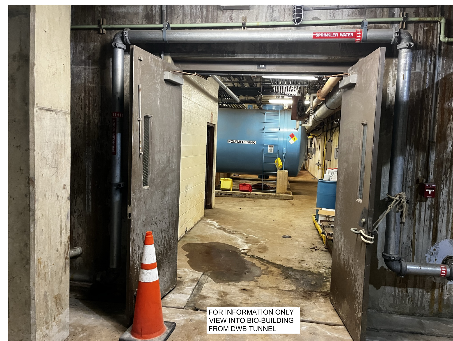
4 DWB TUNNEL-SOUTH WALL M-002
