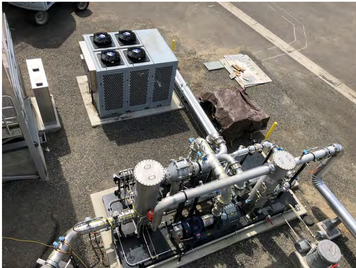
Figure 2. Moisture Removal Installation Example
