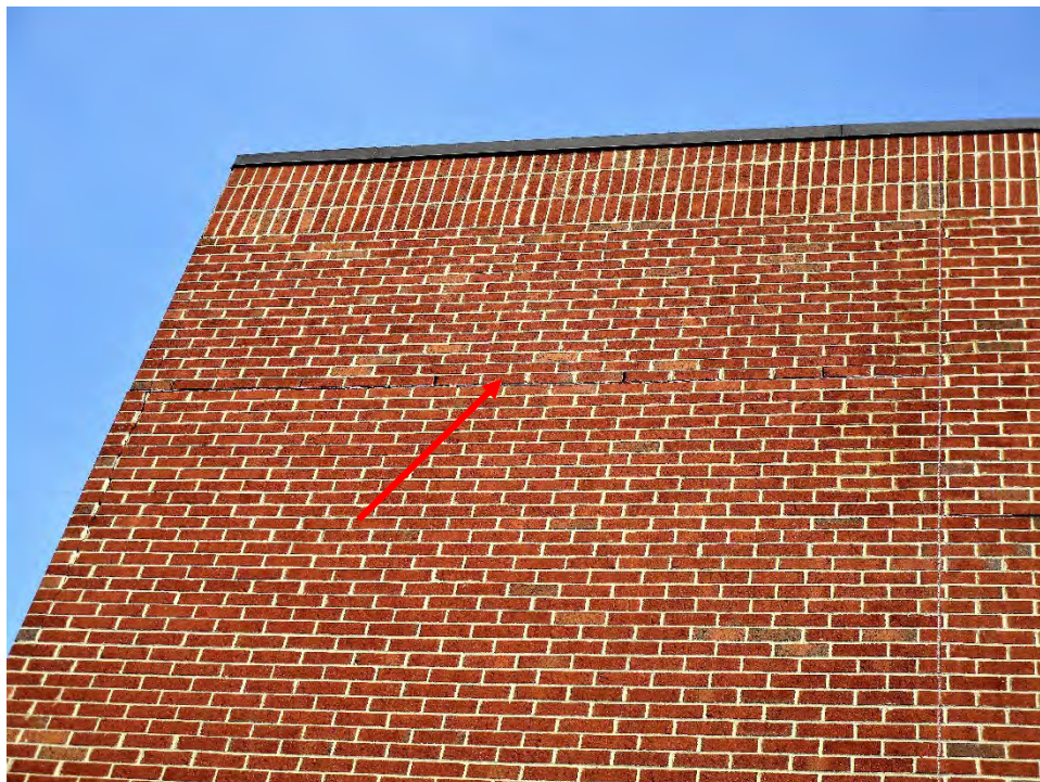
Photo A-45. Brick Joint
