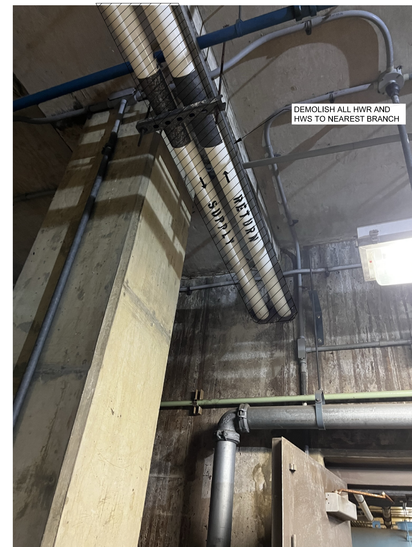
2 DWB TUNNEL-UPPER SOUTH WALL M-002
