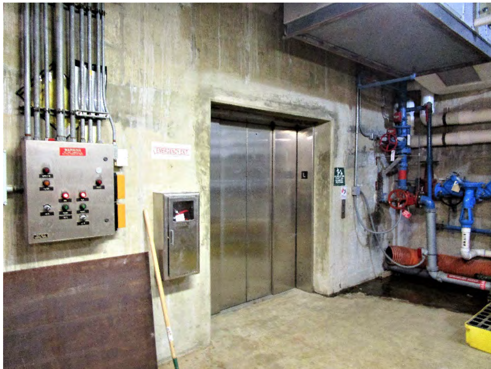
Photo A-31. Save Basement Link to South
