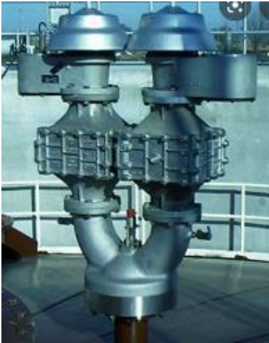
Figure 12-7. PVRVs and Pressure Relief Manhole Cover
