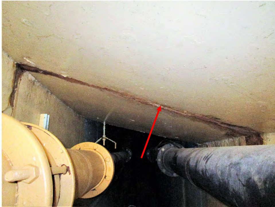
Photo A-25. Joint Needs Investigation
