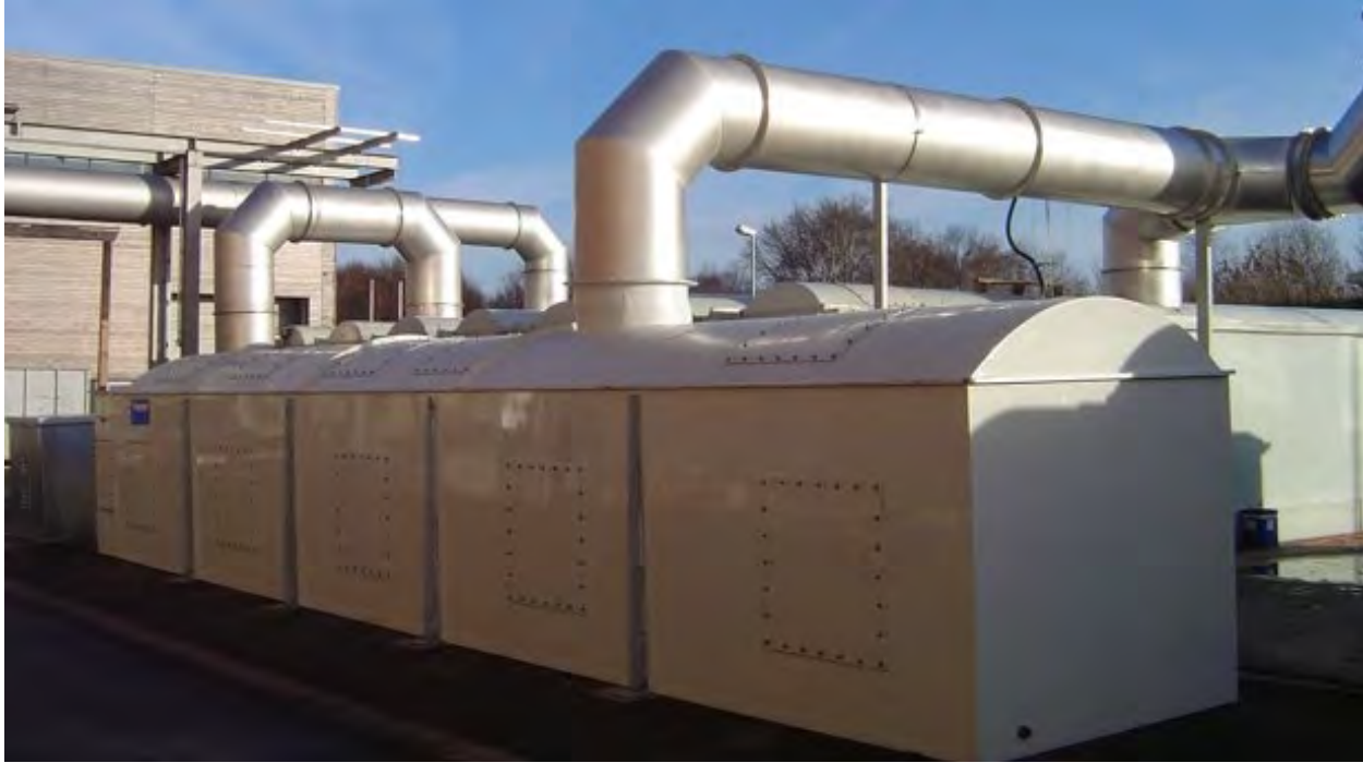
Figure 5. Carbon Adsorption System
