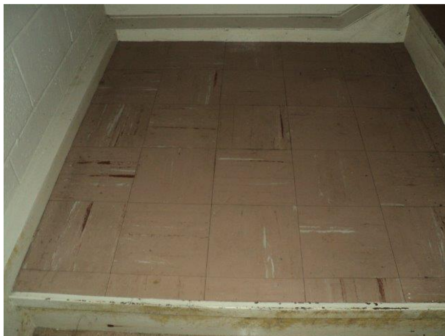
Homogeneous Material No. 7 –ACM 9” by 9” brown vinyl floor tile with black mastic located in the West Side of the Building Stairwell of the Subject Property
