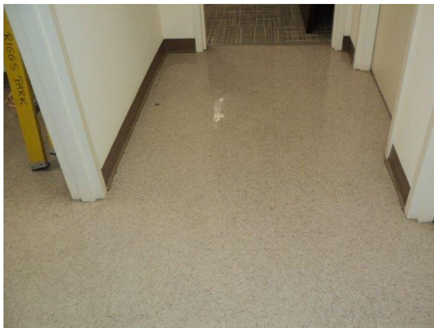
Homogeneous Material No. 12 – Non-ACM 12” by 12” Gray Mottled Vinyl Floor Tile with Tan Mastic located in Building Main Floor, Flooring in Office Area on West Side of Building of the Subject Property
