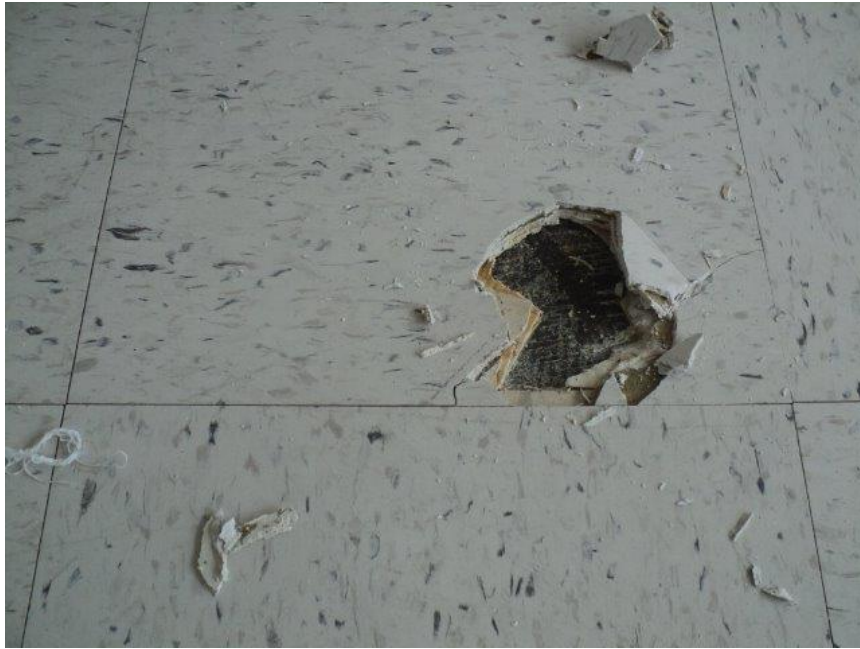
Homogeneous Material No. 23 – ACM 12” by 12” Gray/Black Specs Vinyl Floor Tile with Yellow Mastic over Gray Vinyl Floor Tile with Black Mastic over Gray Vinyl Floor Tile with Yellow Mastic over Cream Resilient Floor Sheet with Black Mastic located in the Building 3 rd Floor Office Space on Northwest Corner
