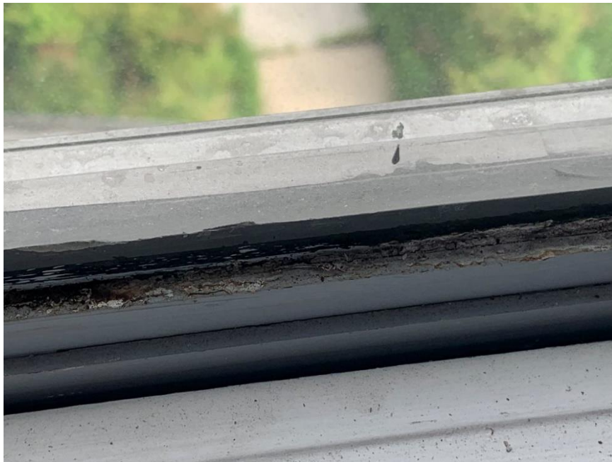
Homogeneous Material No. 24 – ACM Gray Interior Window Glazing Located in the interior windows on the 3 rd floor and throughout the building of the subject property
