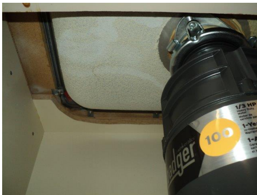
Homogeneous Material No. 14 – Non-ACM Gray Sink Bowl Coating located in the Building Main Floor, Break Room on West Side and on Building 2 nd floor, Break Room on East Side of the Subject Property
