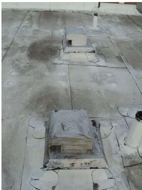
Homogeneous Material No. 3 – ACM Silver Roof Vent Coating located on the roof of the Subject Property
