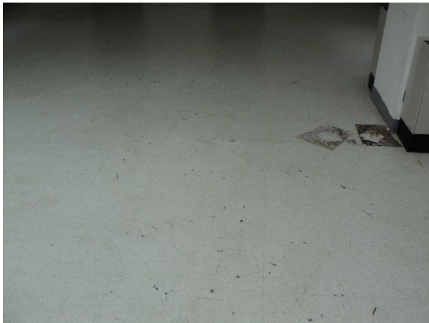
Homogeneous Material No. 19 – ACM 12” by 12” White Mottled Vinyl Floor Tile with Black Mastic and Gray/White Leveling Compound located throughout the Building 2 nd Floor Office space of the Subject Property
