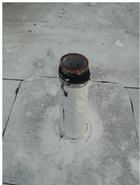
Homogeneous Material No. 4 – Non-ACM Black Vent Pipe Mastic located in the roof of the Subject Property
