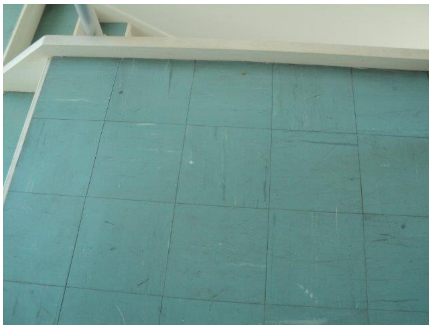
Homogeneous Material No. 20 – ACM 9” by 9” Green Vinyl Floor Tile with Black Mastic located in the building stairwell on East Side
