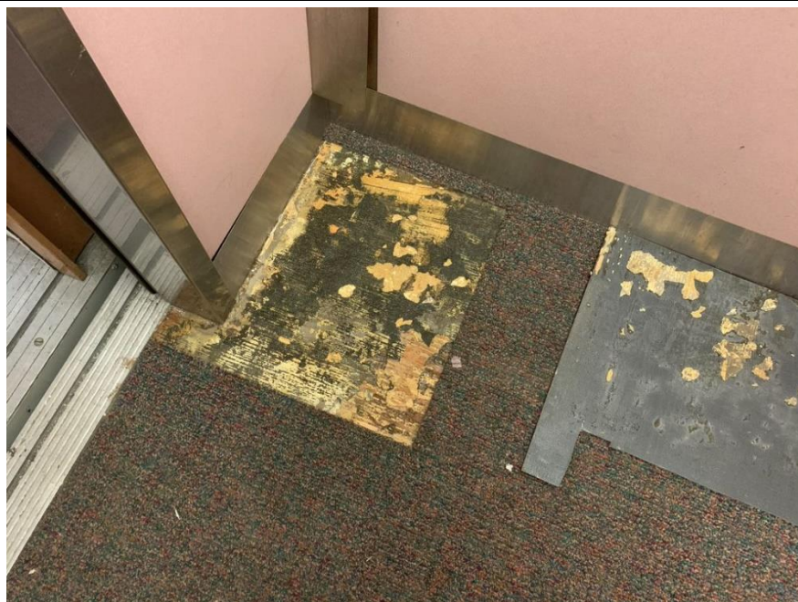
Homogeneous Material No. 9 – Non-ACM Black/Gray/Yellow Mastic located in the Building Elevator of the Subject property
