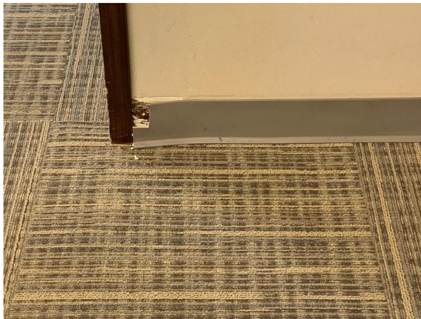
Homogeneous Material No. 15 – Non-ACM 4" Brown Vinyl Cove Base with Brown Mastic Located in the Building Main Floor, Flooring in Some of the Office Area on West Side of Building and Central Customer Area of the Subject Property
