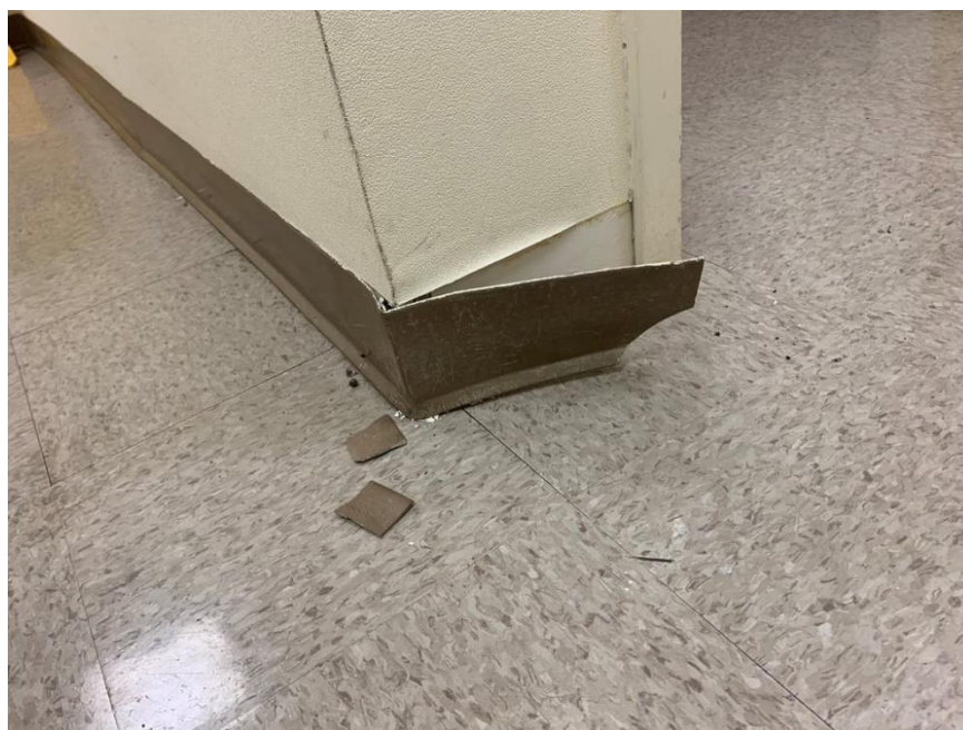
Homogeneous Material No. 13 – Non-ACM 4" Gray Vinyl Cove Base with Gray Mastic Located in the Building Main Floor, Flooring in Office Area on West Side of Building of the Subject Property
