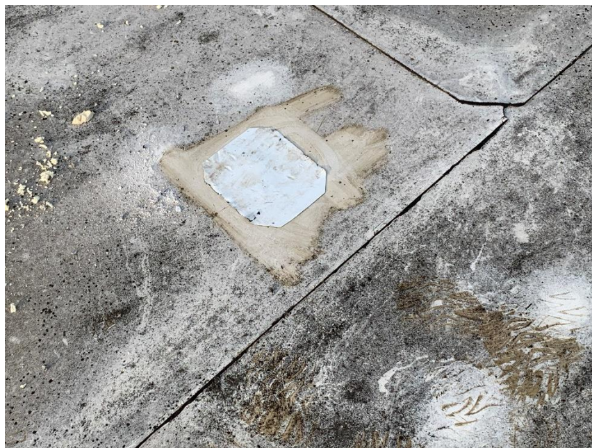
Homogeneous Material No. 1 – Non-ACM Built up Roof Field located on the roof of the Subject Property
