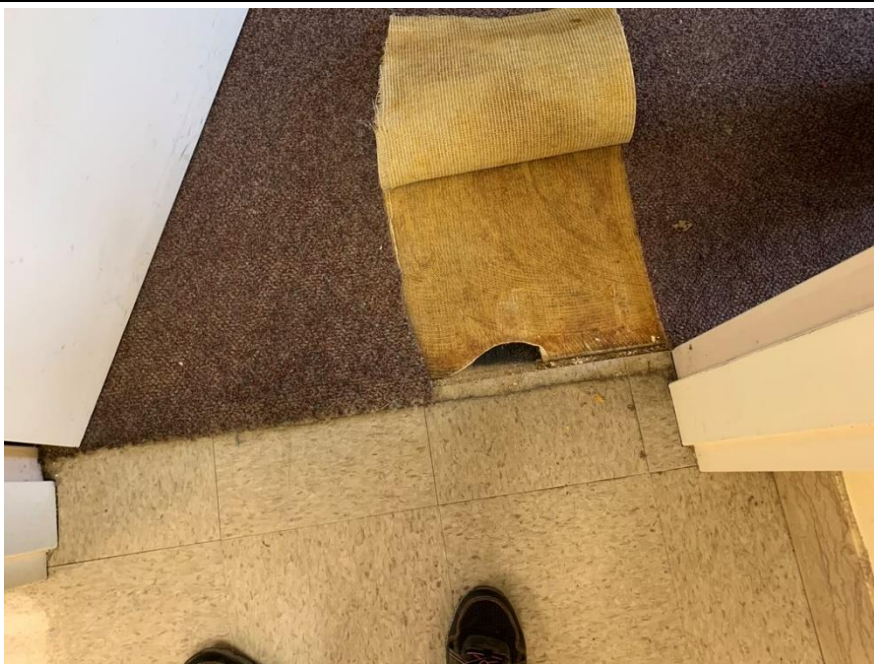
Homogeneous Material No. 10 – ACM Gray Pebble Pattern Resilient Sheet Flooring over Brown Vinyl Floor tiling with black mastic located in Building Main Floor, Corridor near Elevator
