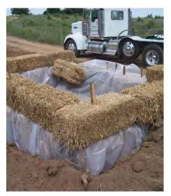
Example washout structures. Note that each example is fully lined and the washout is contained.
