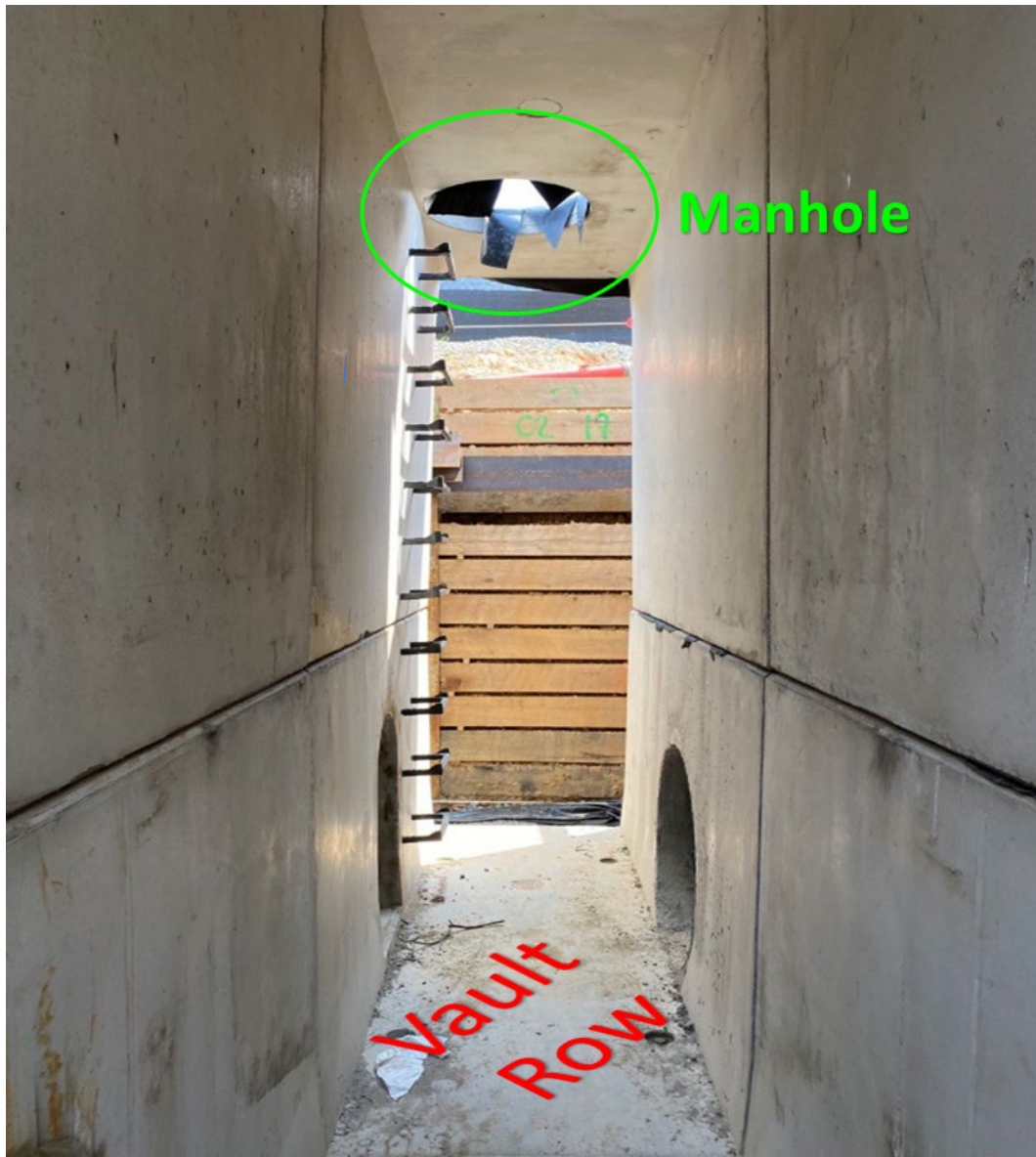
Figure 4. The underground detention vault access manhole
