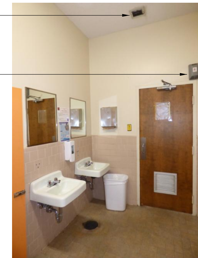
EXISTING WOMEN'S RESTROOM
