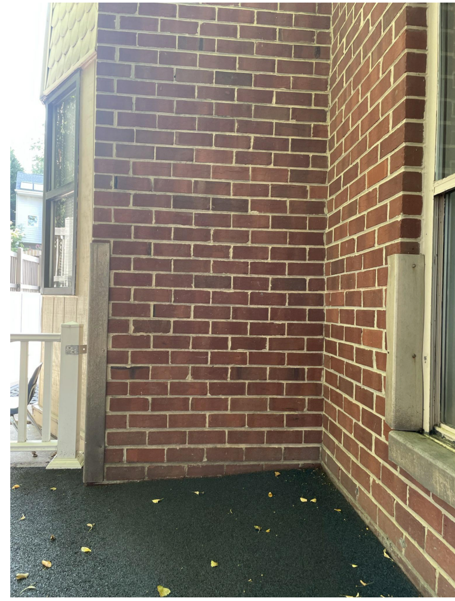
D1/AD103 - DEMO BRICK SECTION
