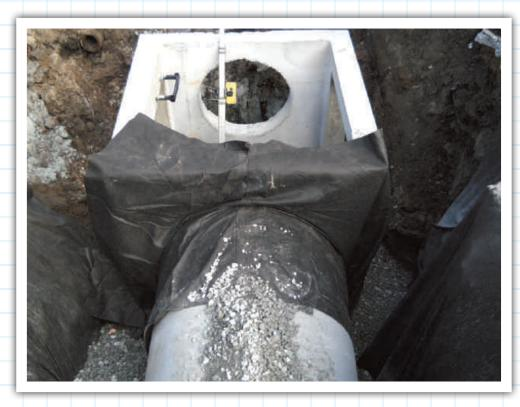
PREVENTS LEACHING AND UNDERMINING OF SUBGRADE MATERIAL THROUGH OPENINGS THAT MIGHT OCCUR AT THE CONNECTION OF THE PIPE AND THE MANHOLE WALL.
