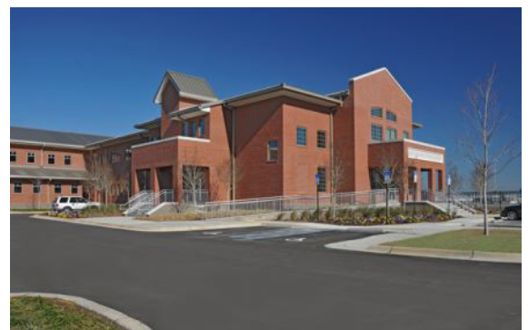
ECUA Administration building at Central Water Reclamation Facility. Mott MacDonald completed the architectural, civil, electrical and structural designs.
