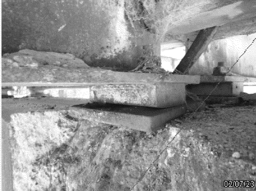
Photo 7: Bearing 19-3 tilting towards the far side causing a gap along near side
