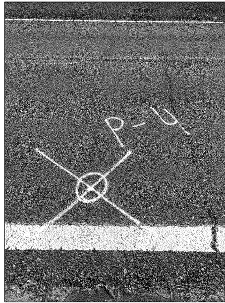
Boring P-4 Located at (30. 917737°, -86.609594°), total thickness of 3 7/8 inches.
