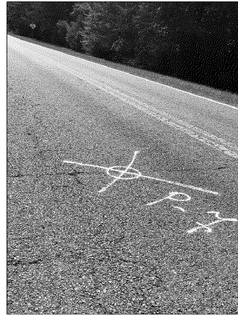
Boring P-7 Located at (30. 925652°, -86. 588494°), total thickness of 3 7/8 inches.
