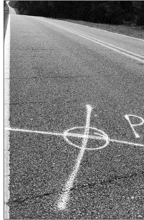
Boring P-14 Located at (30. 924897°, -86. 531723°), total thickness of 4 3/8 inches.
