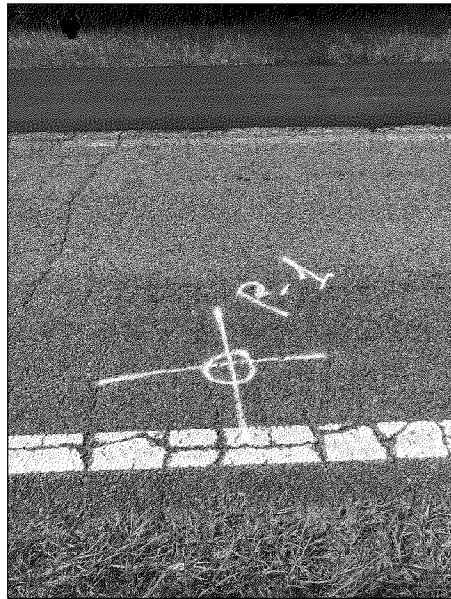
Boring P-1 Located at (30.924767°, -86.632324°), total thickness of 2 3/4 inches.
