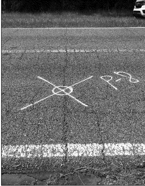
Boring P-8 Located at (30. 925499°, -86. 580349°), total thickness of 3 ¼ inches.
