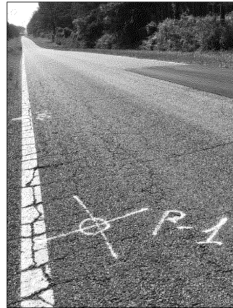
Boring P-1 Located at (30.924767°, -86.632324°), total thickness of 2 3/4 inches.
