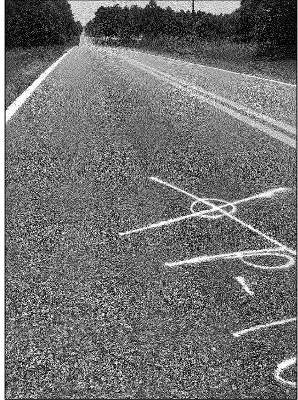
Boring P-16 Located at (30. 924669°, -86. 515431°), total thickness of 2 ¾ inches.
